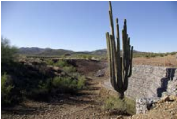
Figure 7.2 Beautiful, large saguaro protected by gabion wall..
