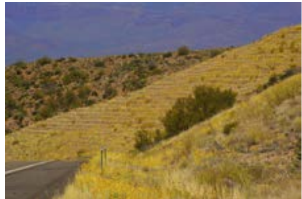
Figure 7.4 Mini benching allows for more water retention thus giving seeds a better chance to take hold.
