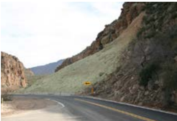
Figure 7.7 Slope on the right has been hydroseeded.
