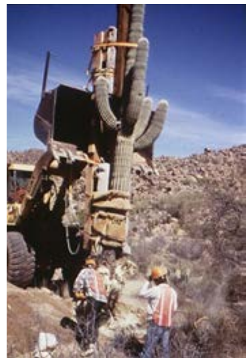
Figure 7.1 Salvaging existing vegetation.
