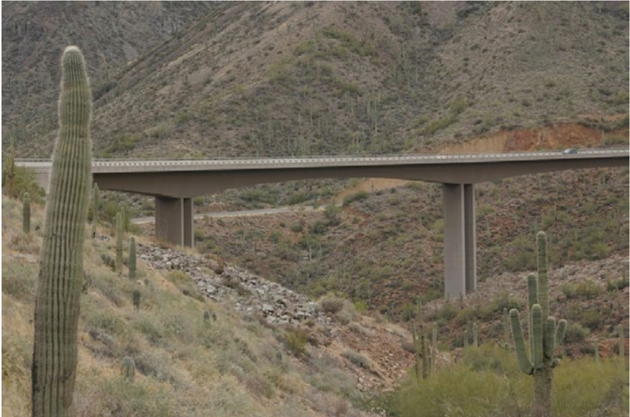
Figure 3.5 With larger dimensions, long spans between bridge supports can have less of an impact on sensitive wildlife corridors while allowing traffic to move overhead.
