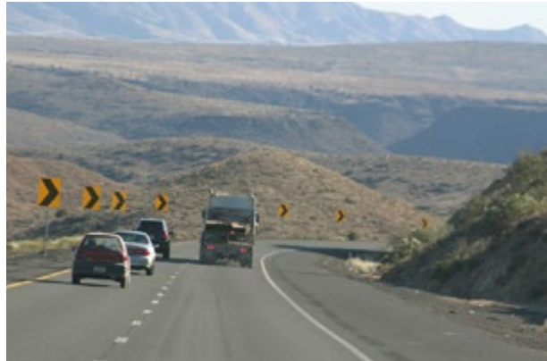
Figure 3.3 Reducing speed by designing with steeper grades.
