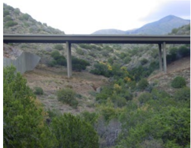
Figure 3.7 Bridge crossing a natural drainage, built high to preserve riparian ecosystem.
