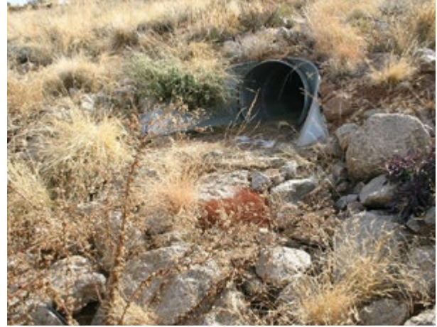
Figure 3.12 Small pipe culvert.
