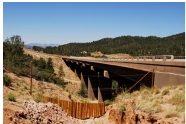
Figure 3.15 Fence designed to facilitate wildlife passage under the roadway.
