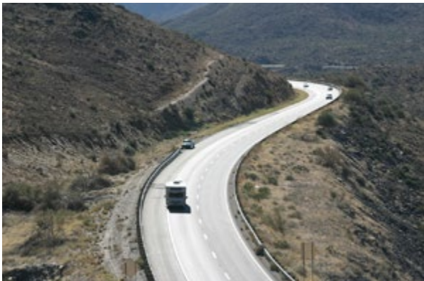
Figure 3.2 Highway laying lightly upon the natural terrain.
