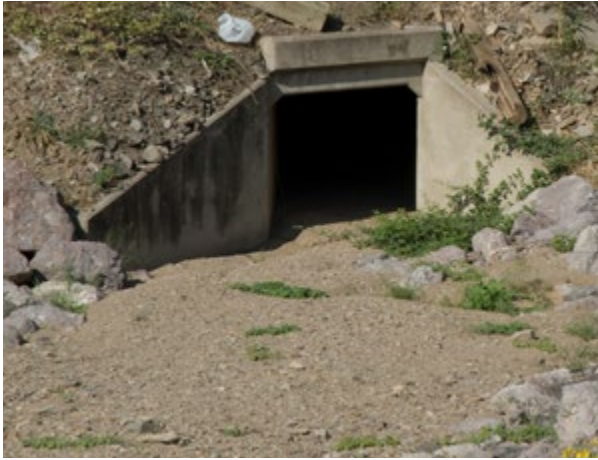
Figure 3.11 Culverts should be free of obstacles.
