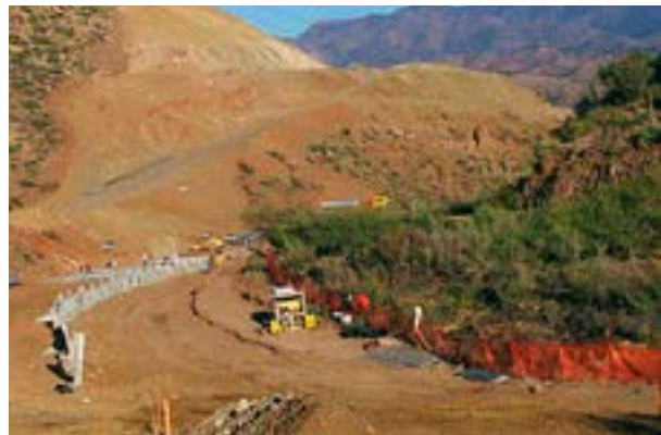
Figure 10.4 Barrier marking materials may be required for areas to be left undisturbed.
