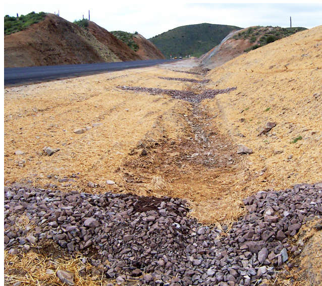
Series of check dams in roadside ditch.
