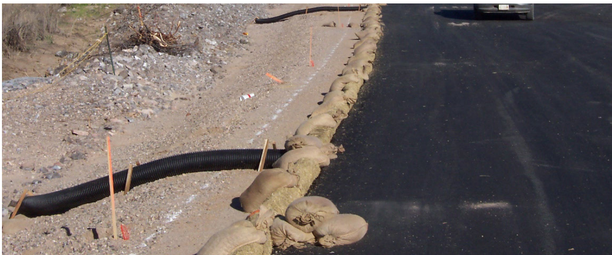
Slope Drain Installed at the edge of impervious pavement to control slope erosion from run on.
