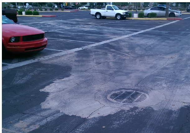
Storm drain inlet has not been protected.
