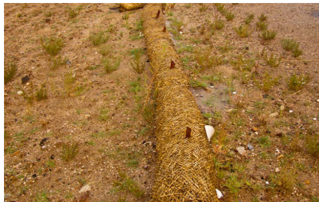
Proper staking of wattles.
