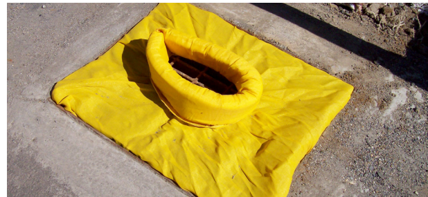
Fabric protections designed to not clog or block a drain are a good application for this drop inlet
