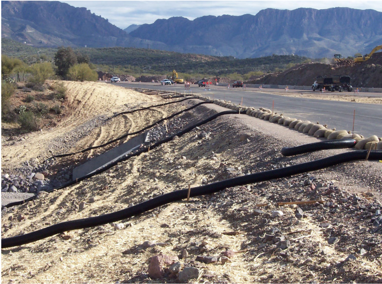
End of slope drains are directed to a stabilized, rock-lined transition ditch.
