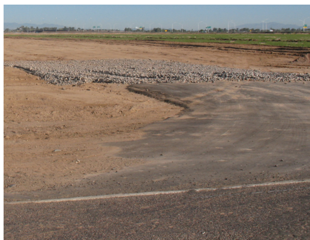
Some jurisdictions will require "cold mix" asphalt to join the gravel pad to the roadway. Coordinate with County and municipalities prior to installing gravel at their edge of pavement.
