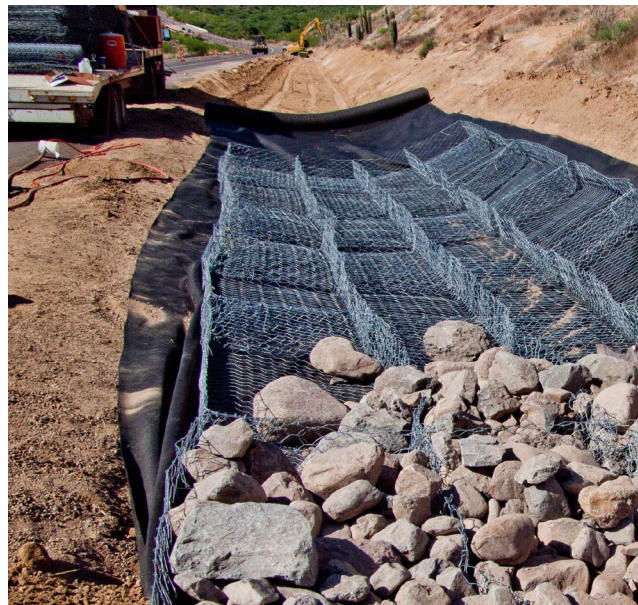
Gabion mattress designed for anticipated high PP velocity flows.
