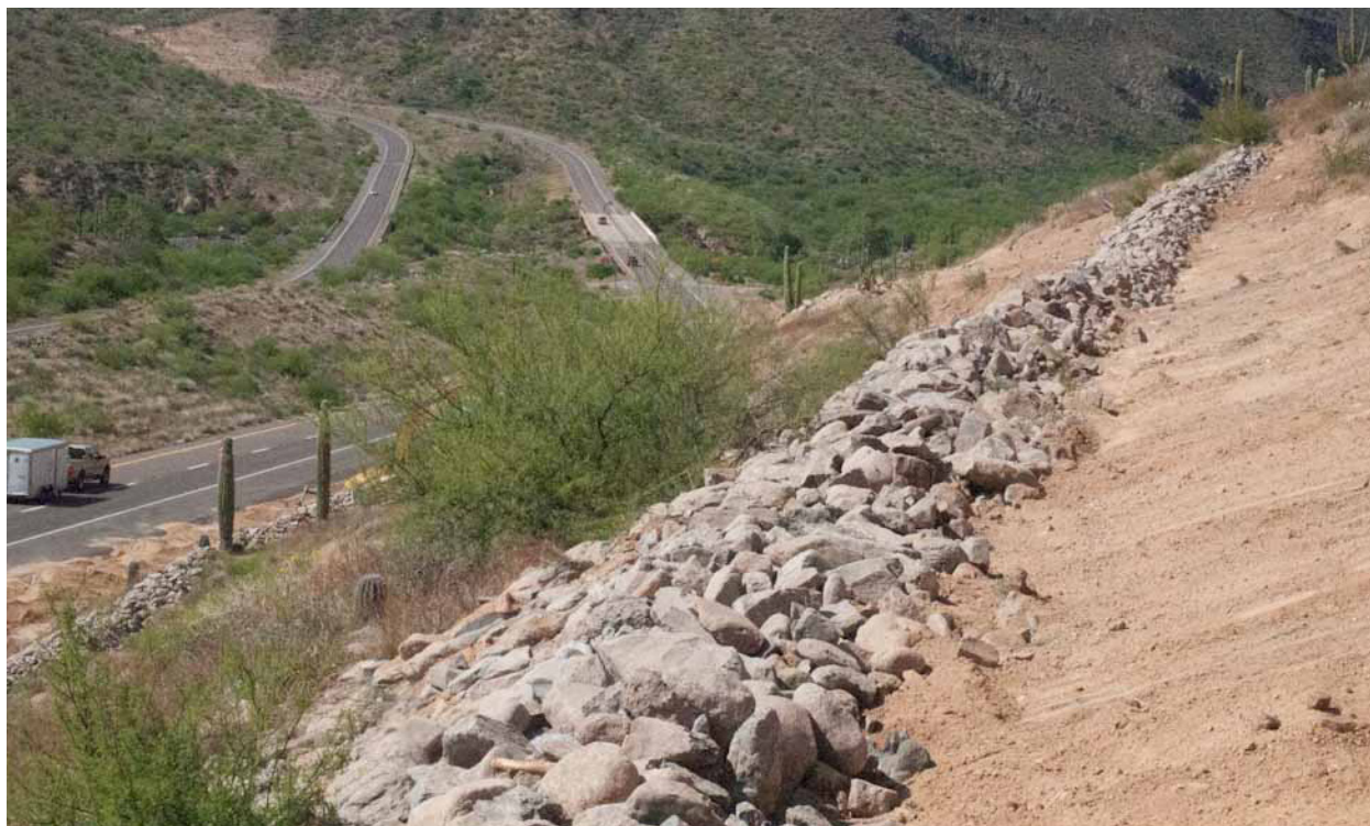
Berms run parallel to slope contours and are trenched into slope face.
