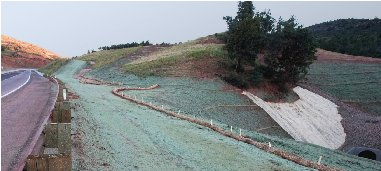
Mature trees preserved in place. Notice sediment wattles, erosion control blanket, seeding and mulch cover Stormwater Control Measures used in combination to achieve the most effective erosion control for these site conditions.
