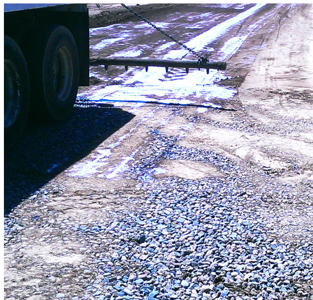
Application of soil binder.
