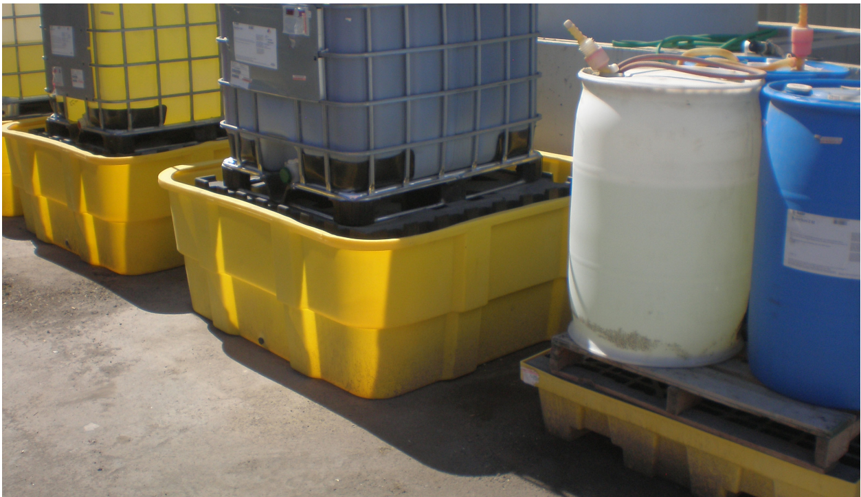
Commercially available containment pallets are designed to meet 40 CFR regulations for drums and totes.
