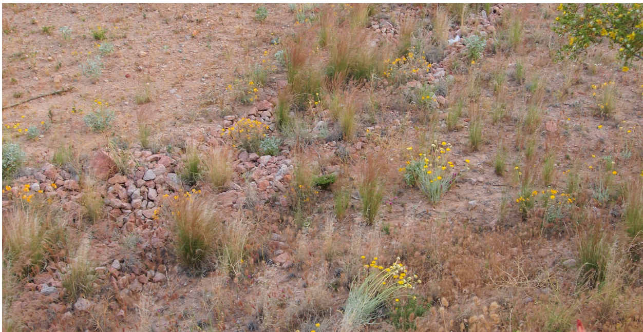
Rock line cut to fill transition ditch properly installed and over-seeded. Riprap should blend with landscape.
