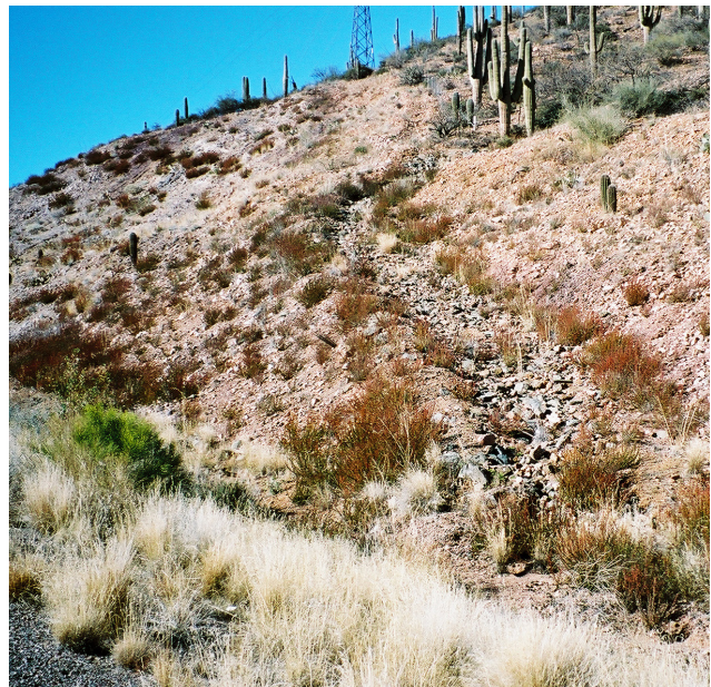
Gabion-style crown ditch used for extreme drainage conditions and slope retrofits.
