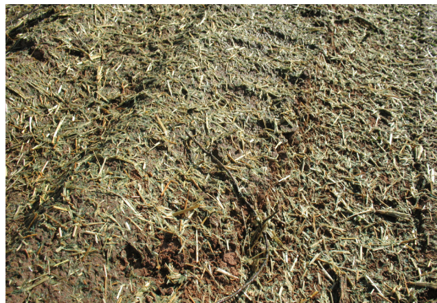
Straw mulch cover used in combination with approved seed mix.
