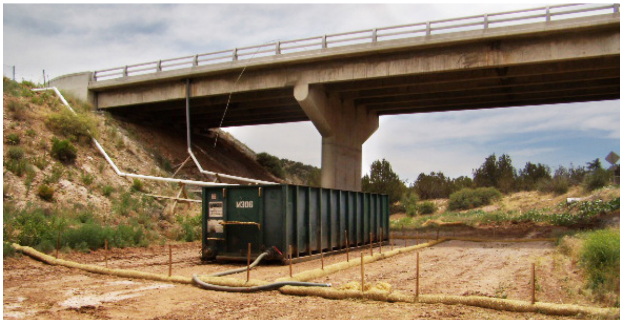
Dewatering during bridge work.
