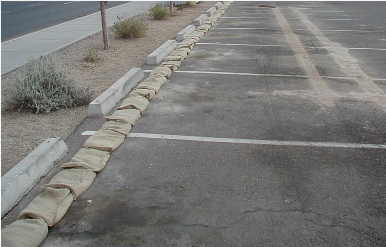
Gravel bag perimeter control for paved areas (where no staking or trenching is possible).
