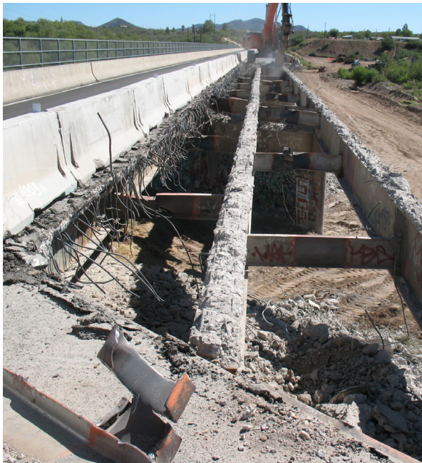
Demolition over the San Carlos River where clean Water Diversion (NS-5) was used to keep the river clean and free of debris.
