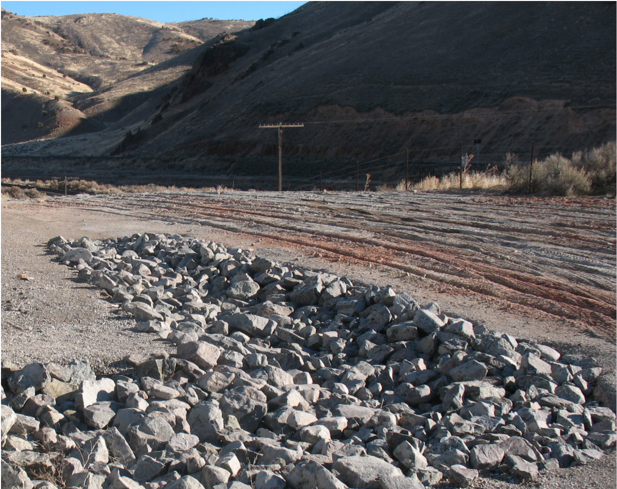
Rock lined ditch installed incorrectly. Rock is not keyed in and stormwater flows will erode the sides, causing failure and rework.
