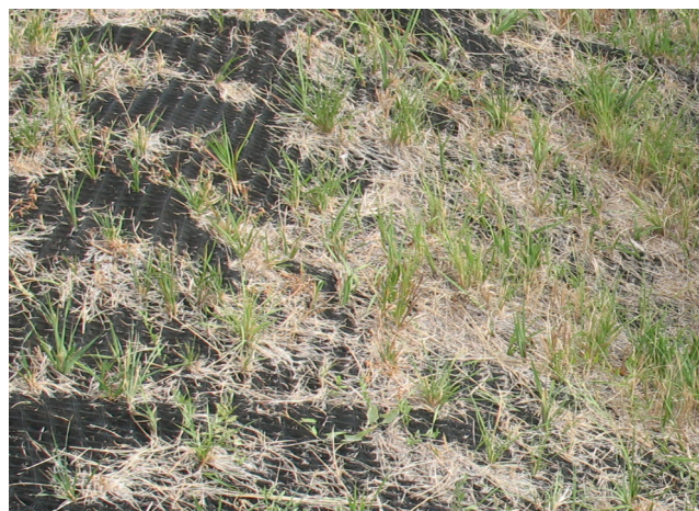
Turf Reinforcement Mat (TRM) - Note vegetation growing through open weave.
