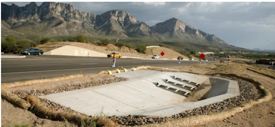
Rock mulch and sediment logs used to protect storm drain inlet.
