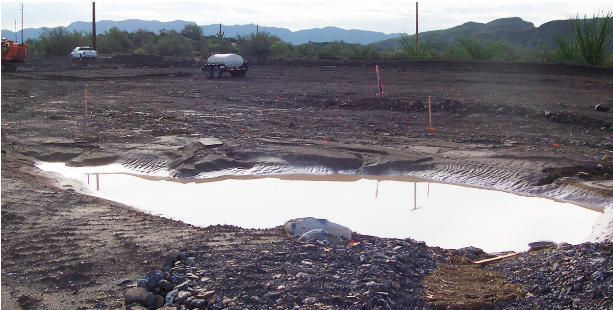
Trap situated to collect sediment laden water prior to discharge.
