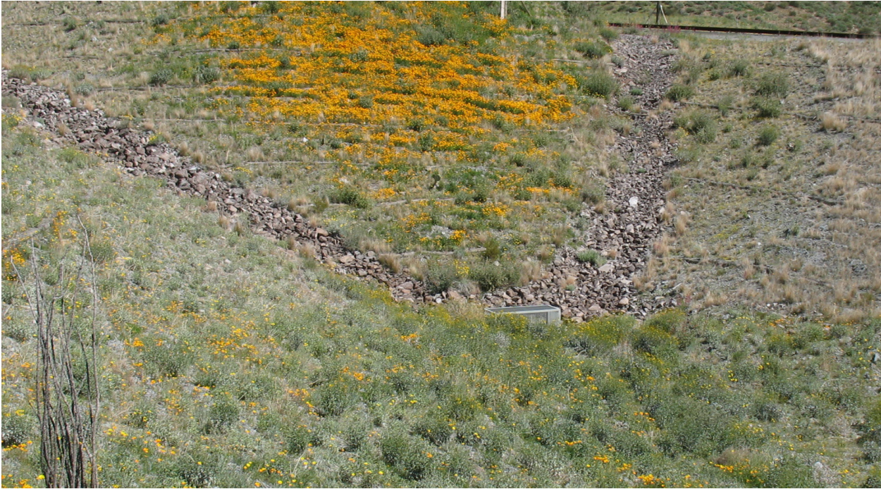
The same drop inlet (different angle) with rock properly installed, protecting structures from erosion and sediment loss.
