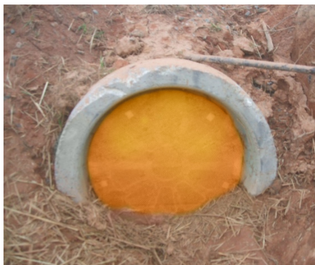
Pipe inlet protection constructed of all mesh (High Flow) to capture large debris and floatable straw mulch.
