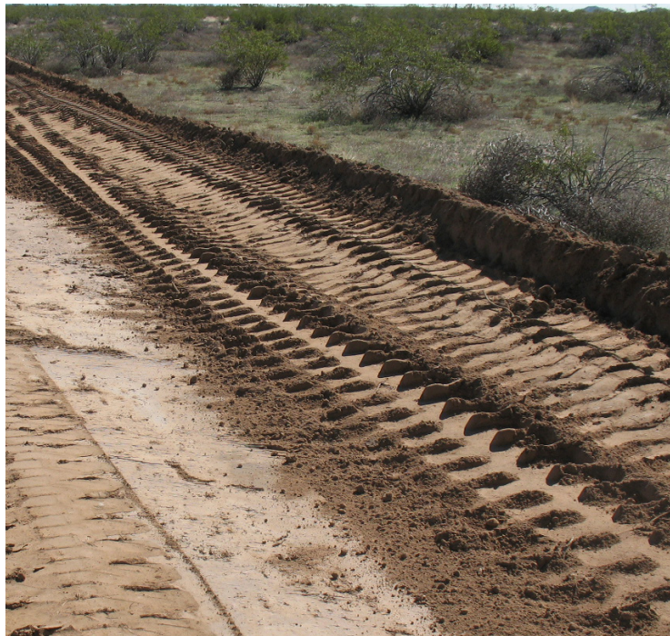
Earthen Dike has compacted berm.
