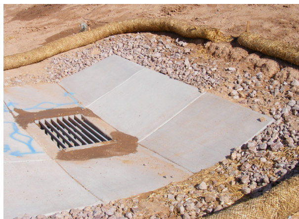
Proper Installation is critical. Logs should be trenched, staked and completely surrounding the rock mulch.
