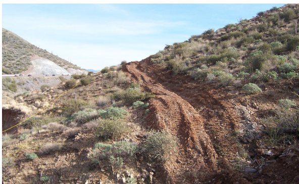
Crown ditch installed early in construction to protect landscape and materials.
