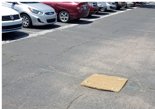
Coir (Coconut fiber) matting has been installed and pavement has been swept.
