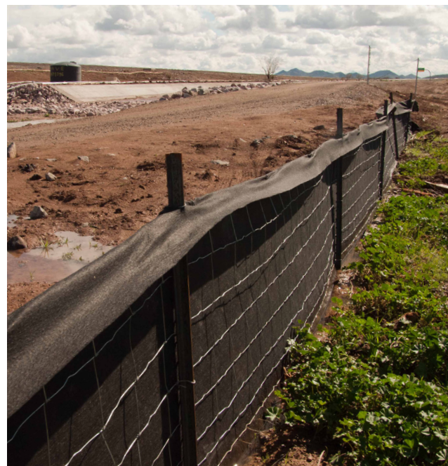
Proper wire mesh support for fabric.
