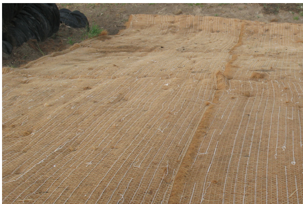
Erosion Control Blanket (coir with plastic netting).
