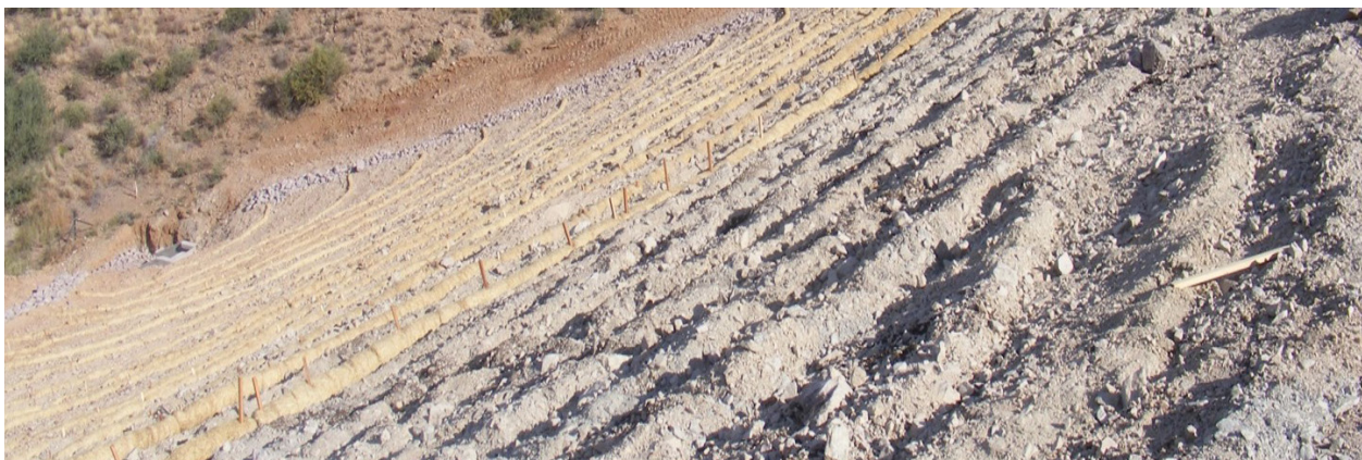
Wattles have been trenched in, staked properly and slope has been roughened prior to installation.
