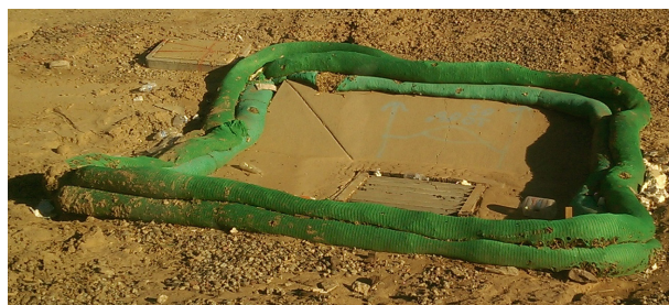
Compost socks are designed to allow for flow and filtration.
