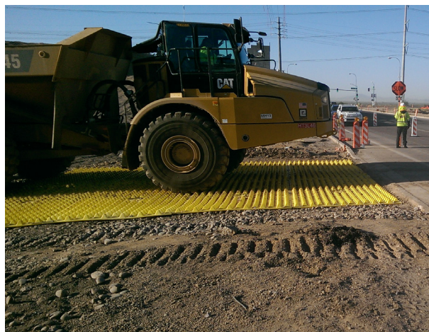
Track mat with gravel pad combination.
