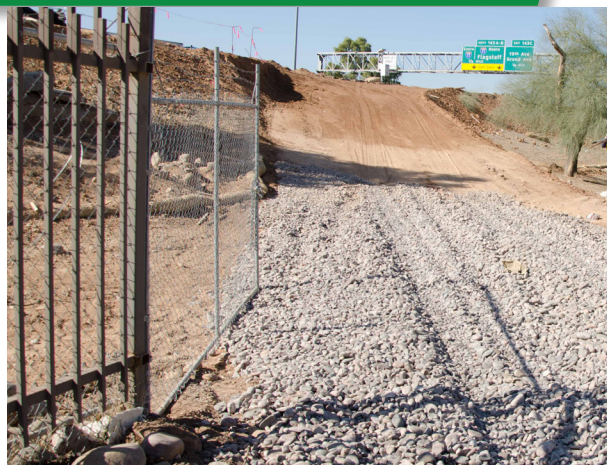
Fencing ensures vehicles enter / exit over the entire length of the trackout device.
