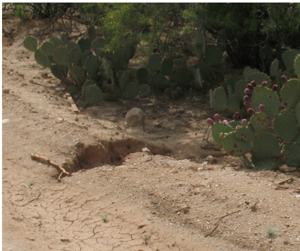
Uncompacted berms will breach and yield a sediment discharge. Sandy soils will not compact well.
