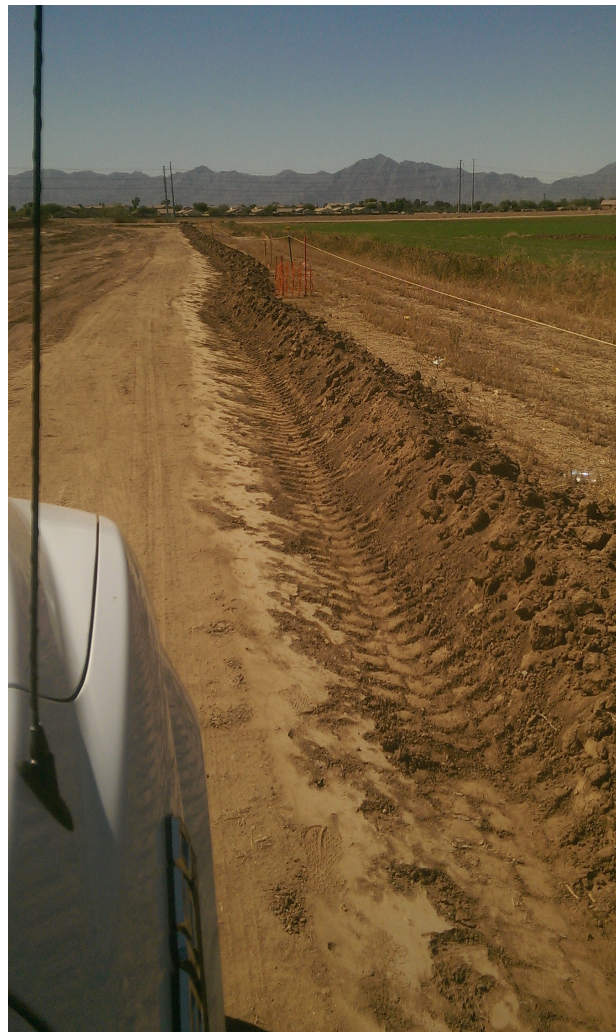
Berm about to be compacted. Will require a stabilized weir and outlet after compaction.
