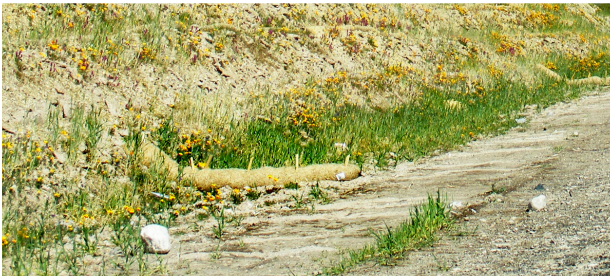
Sediment Wattle Check dam.
