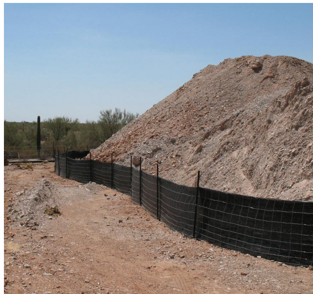
Larger stockpiles in storage yard, surrounded with silt fence and covered with bonded fiber matrix.
