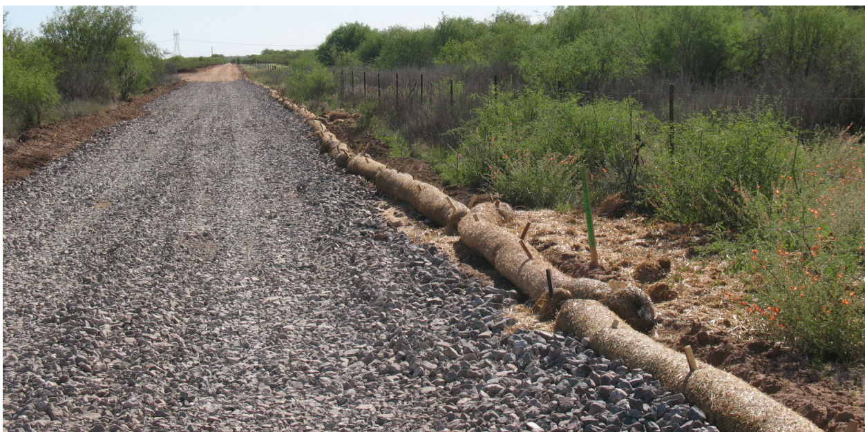
Aggregate-stabilized roadway.
