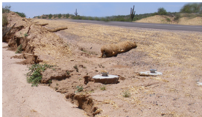
Sediment logs used as check dams. Notice the last log has become dislodged due to poor staking.
