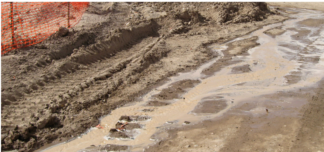
Uncontrolled cleaning water can cause sediment discharges and trackout problems.
