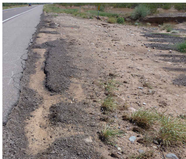
Millings on slight slopes may wash away and increase erosion and run off.
