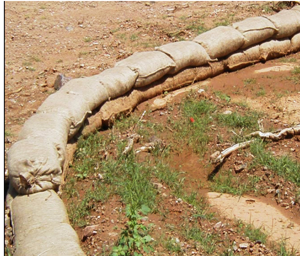
Notice the sediment and water retention held on site (no discharge) allowing seeding to establish quickly.
