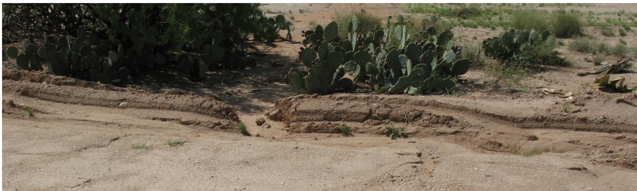
Sediment Berms that are not compacted will lead to failure.
