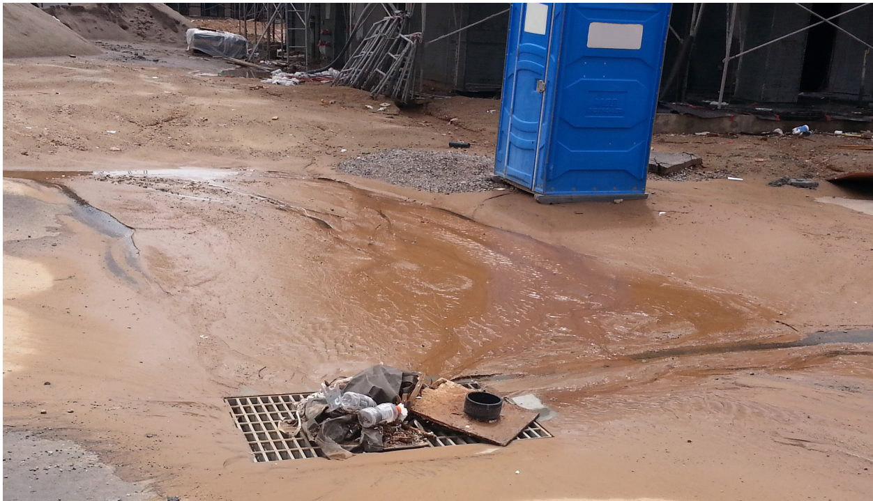
Sanitary facilities require a position at least 100 feet away from water conveyances and storm drain entrances. No other stormwater control measures are present in this photo.
