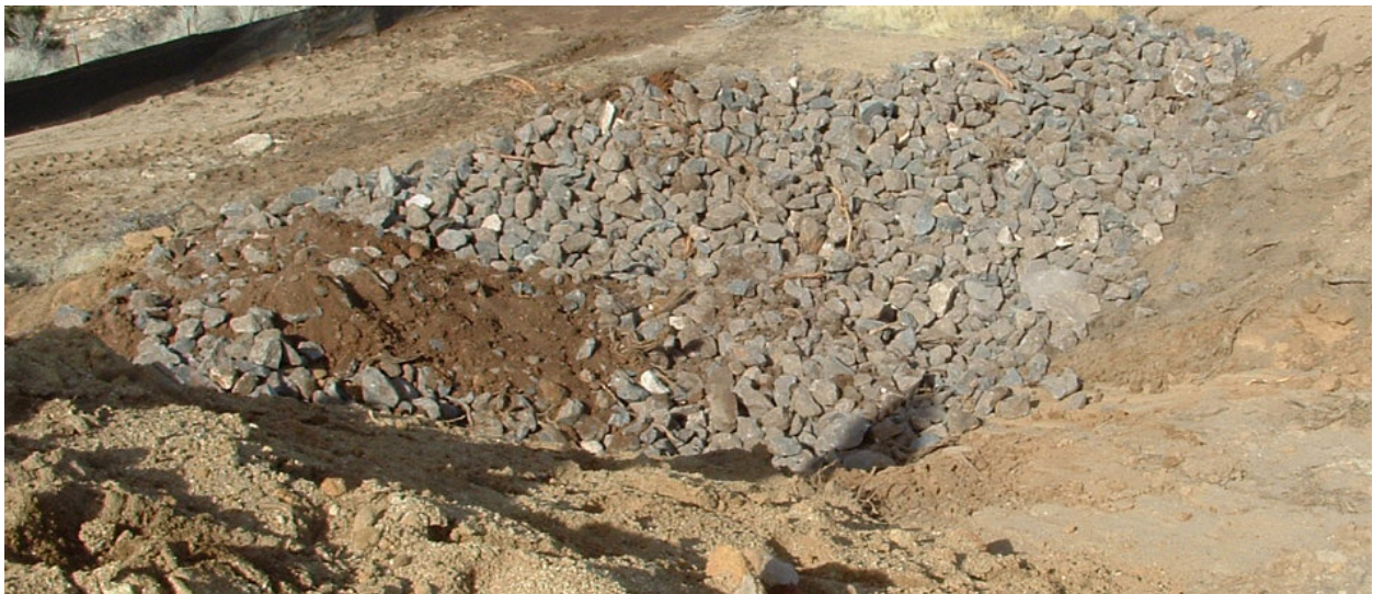
Small, rock-lined sediment trap installed prior to the project boundaries, where overland flows concentrate and may discharge off-site.
