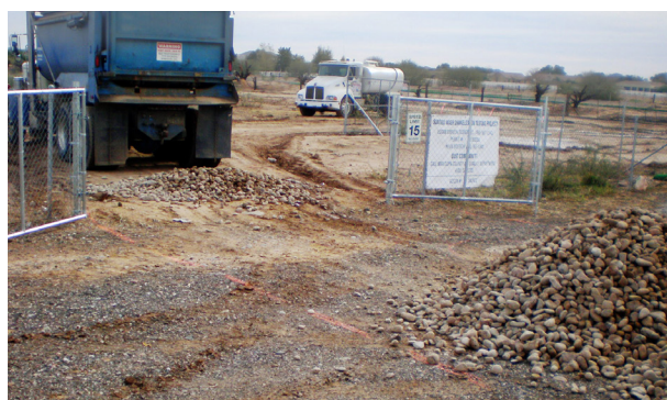
This rock is round "river-rock". Ensure track rock is per specification prior to delivery. Once the truck tilts, you own it.
