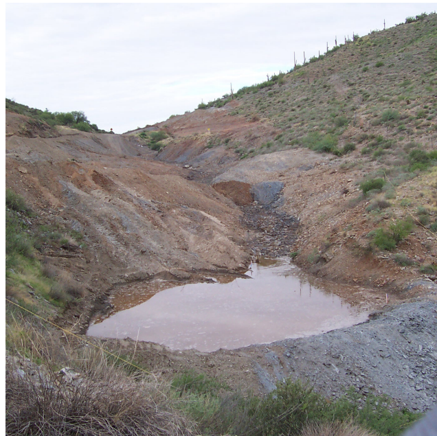
Basin is too small to provide adequate retention for acres drained. A stabilized outlet is required.
