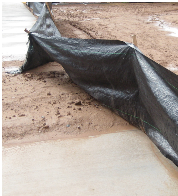
Silt fence has no wire mesh, not trenched in, did not use T-Post, and is installed on the wrong side of the flow.
