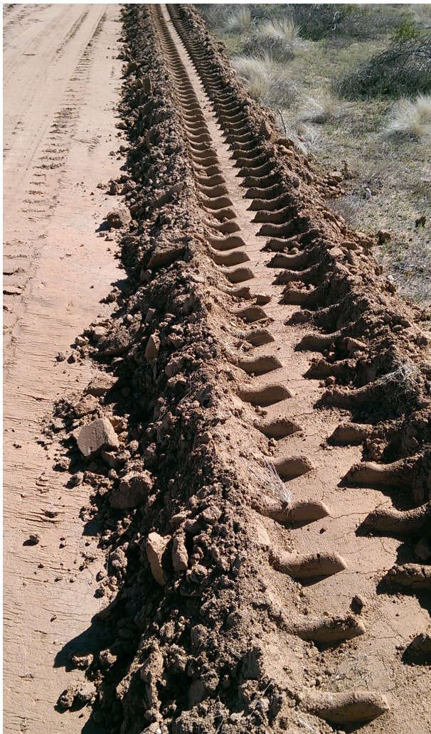
Fully compacted berm protecting surrounding undisturbed areas
