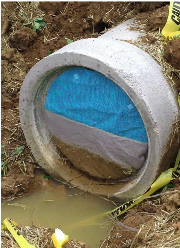
Sediment has accumulated at the filtration section and prevented sediment loss. Pipes must be clean prior to acceptance by ADOT.
