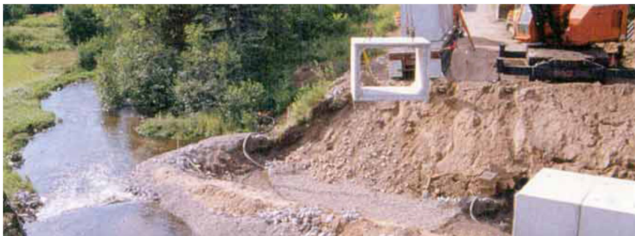
A flow bypass channel is used during placement of a multi-section culvert. Note the clear water in the diversion channel.
