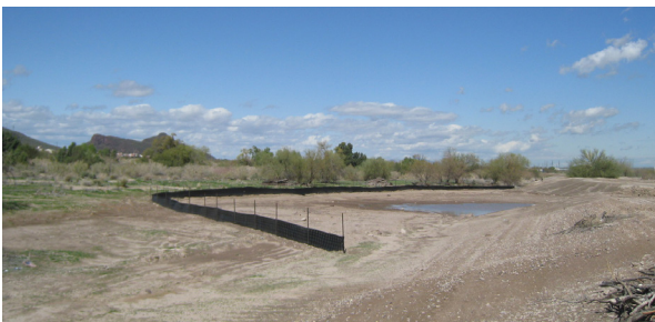
A large area allows sediment to settle out.
