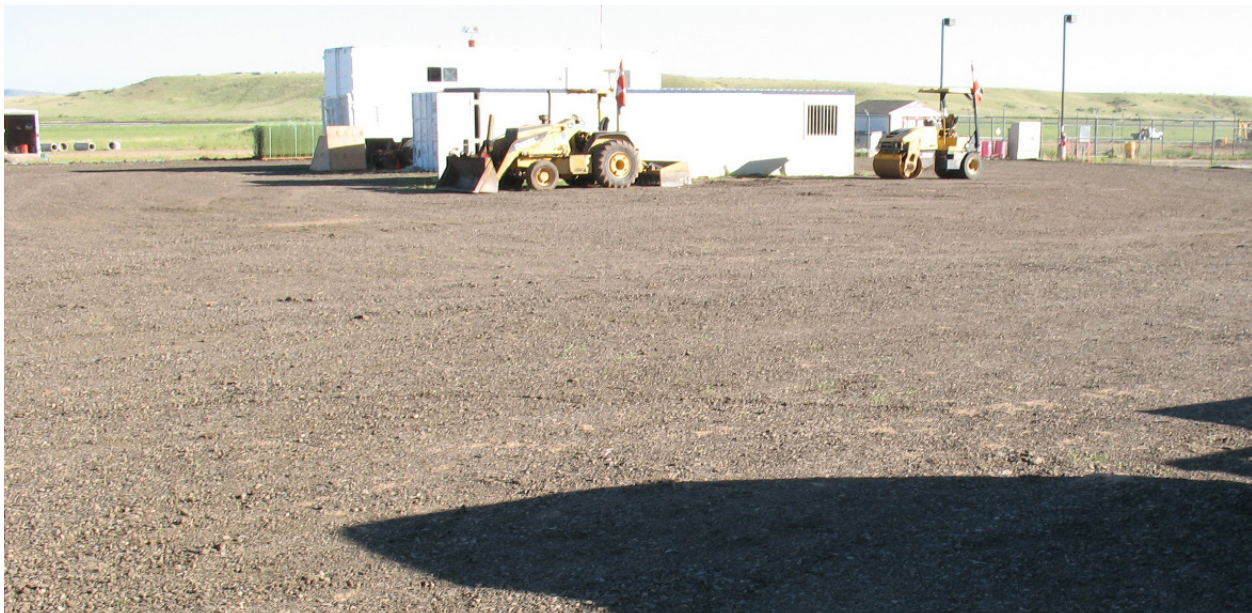
Proper rock cover application on relatively flat soils to prevent wind and stormwater erosion at a construction laydown yard.
