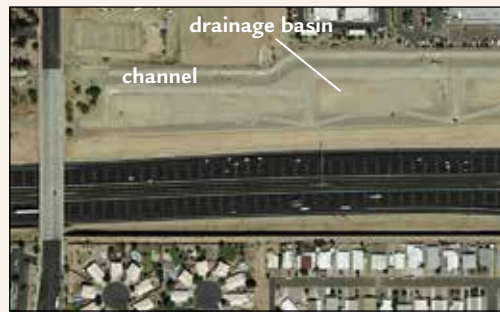
Narrow parallel retention basin
