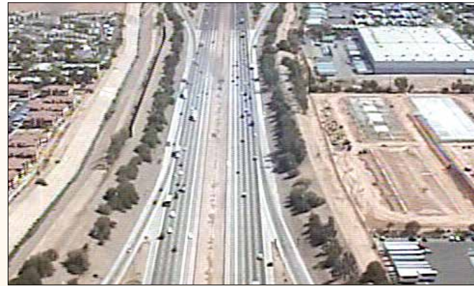
(b) I-10 at 71st Avenue, looking east
