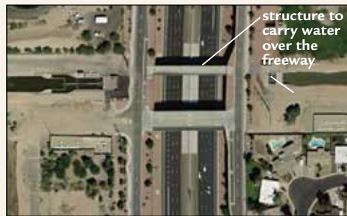
Channel over freeway
