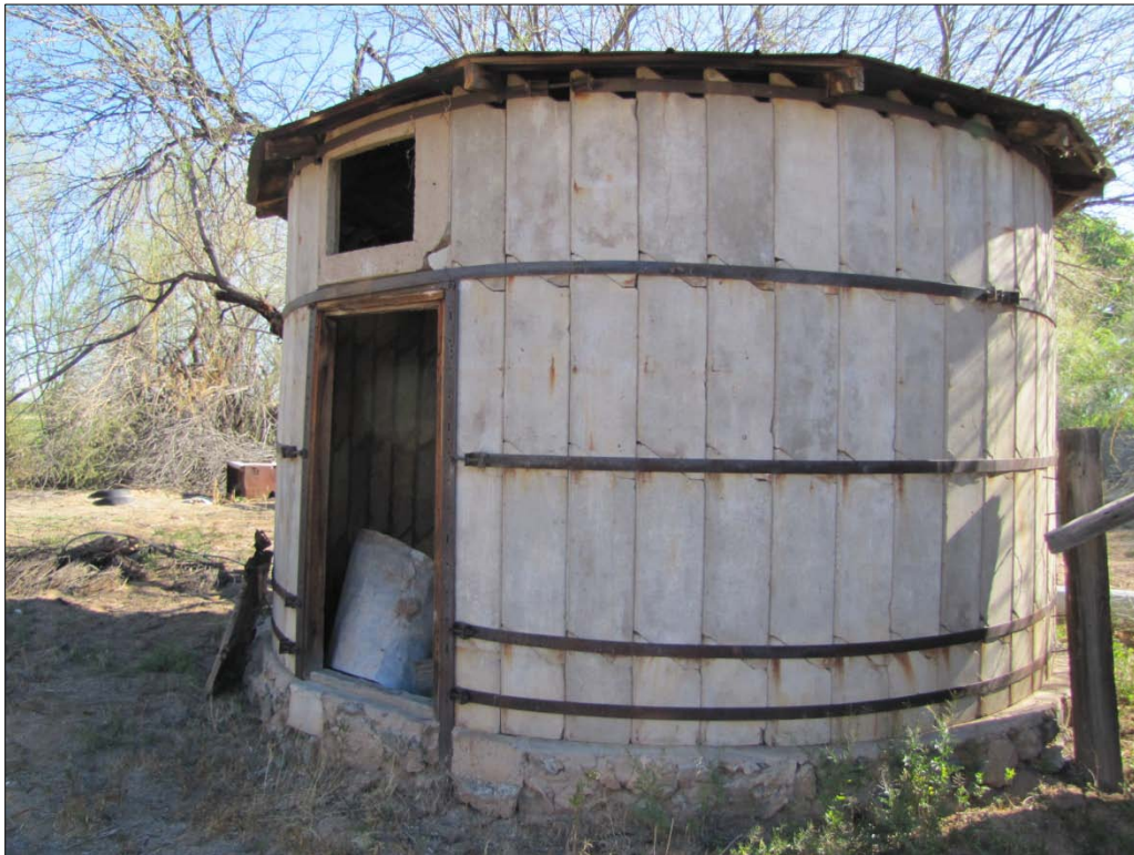
Figure 14. A cement stave silo on the Hudson Farm (Inventory No. 1.03).
