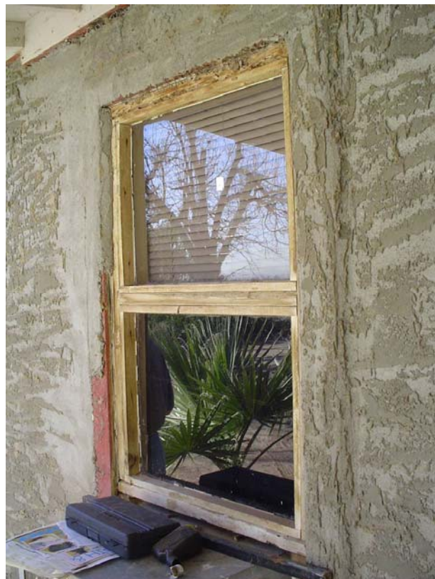
Improper application of stucco to window surround on main house, looking east.
