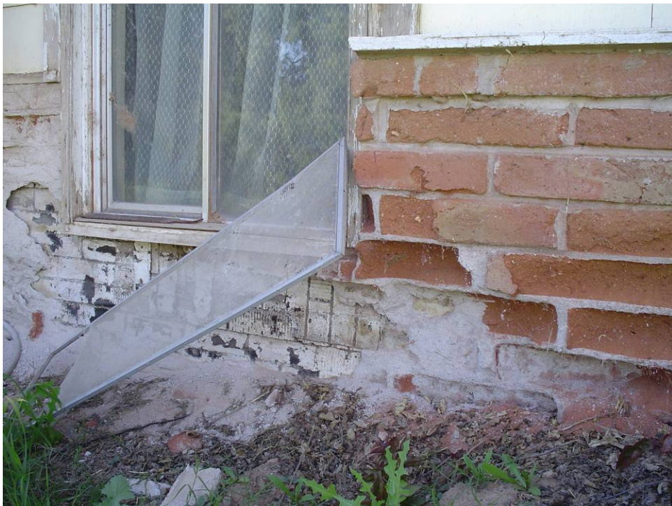
Detail of deteriorated exterior veneer on east facade, looking northeast.
