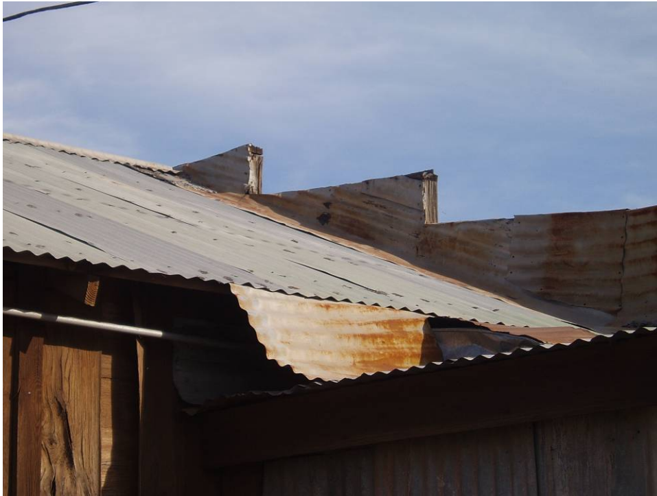
Detail showing rear of false parapet and metal roof at juncture of original building and sheet metal addition on southwest corner, southeast.
