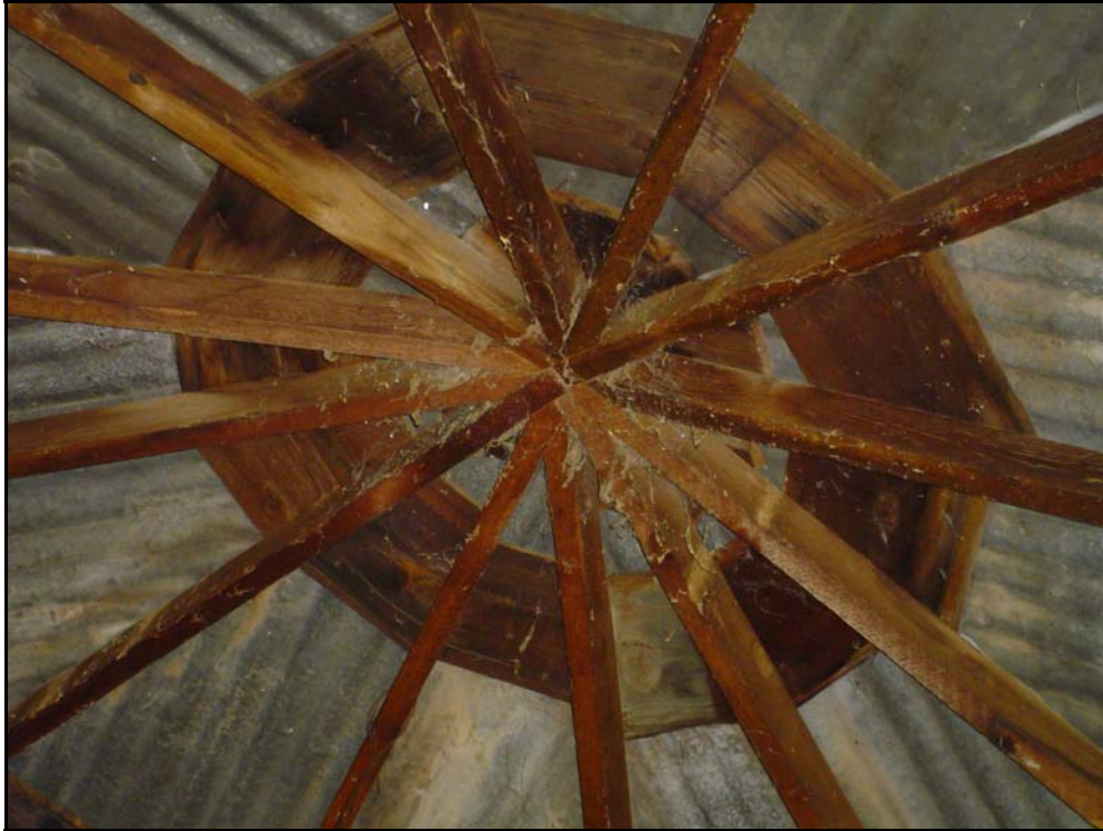
Figure 6.78. Hudson Farmstead: stave silo, interior roof structure.
