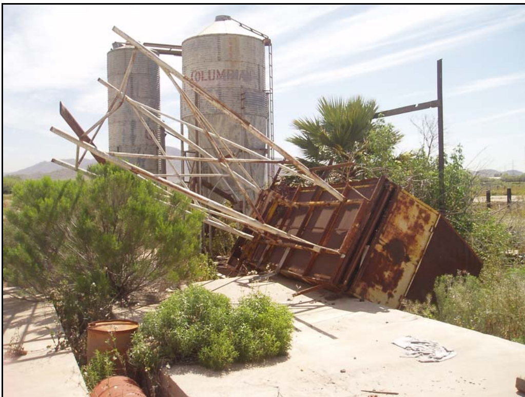
Figure 6.48. Pitrat Feedlot: silos, toppled elevated grain bin, and concrete holding tanks.
