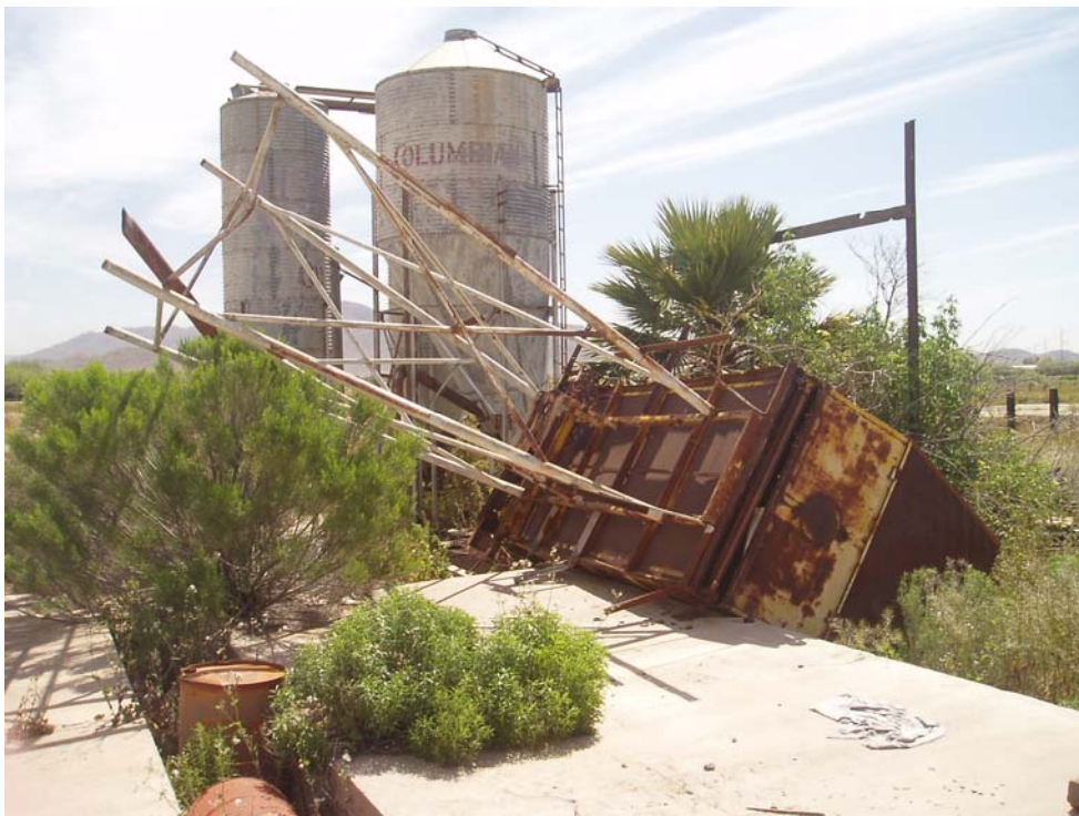
Toppled, elevated grain bin, looking east.
