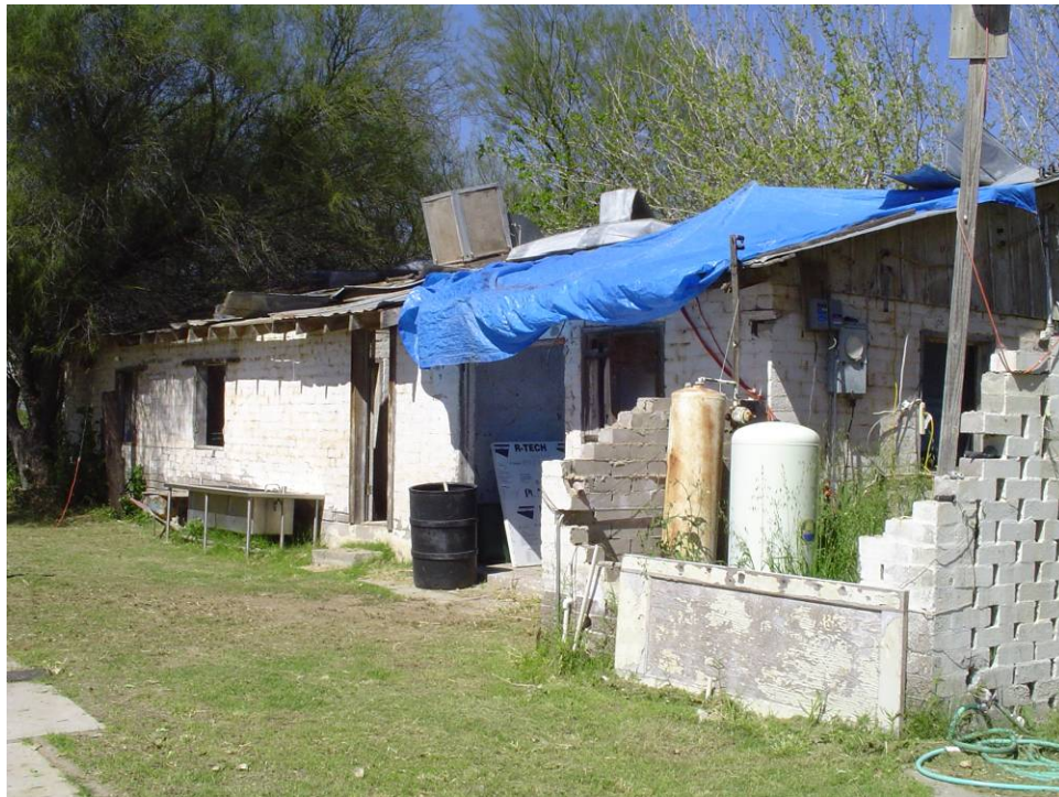
South façade of dairy flat barn, showing deteriorated roof, looking northwest. Dry-stacked concrete block to right of photo is temporary enclosure for propane tanks.
