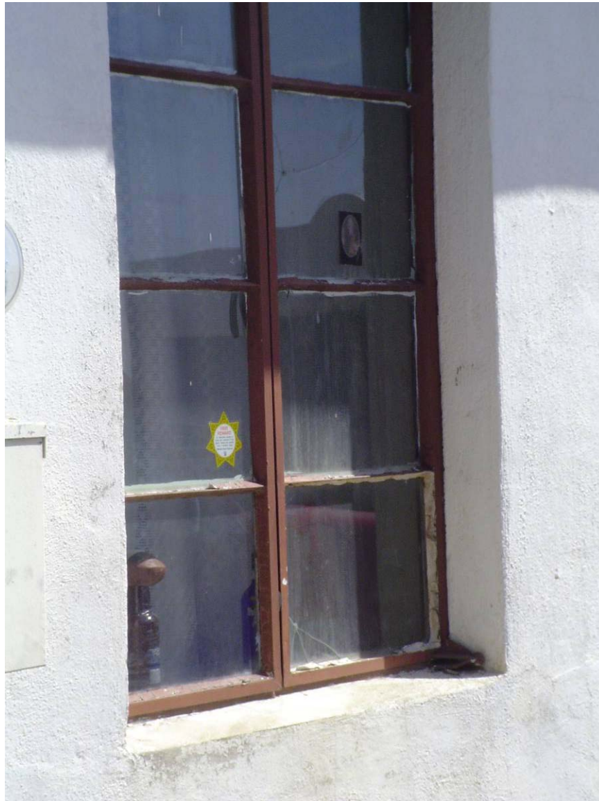
Eight-pane metal casement windows, west façade of 9901 residence, looking southeast.
