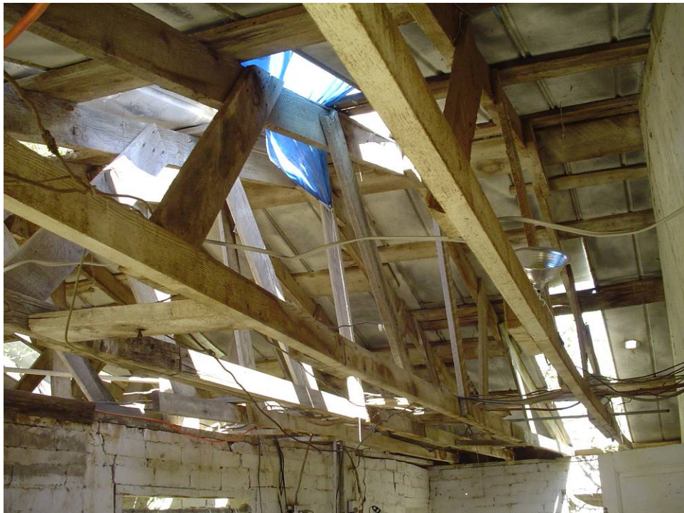
Wood roof truss system in west (milking) room of flat barn, looking southeast from double sliding cattle entrance doors.
