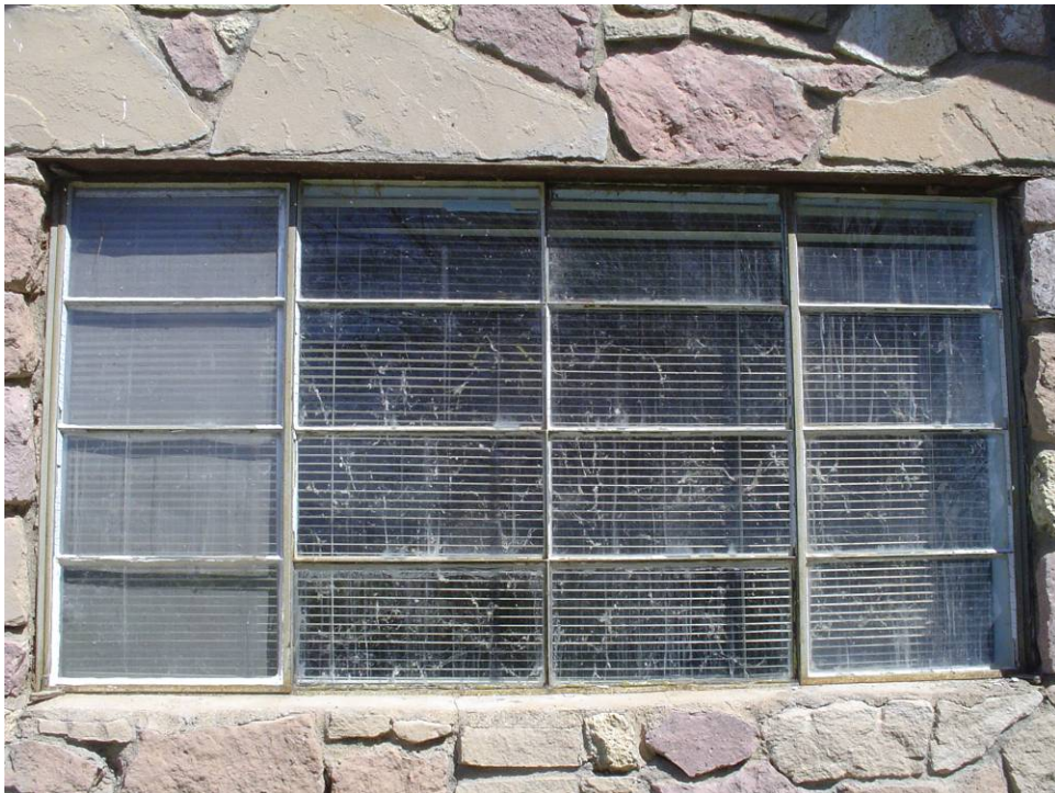
Metal casement windows system on south façade of main portion of house, looking north.
