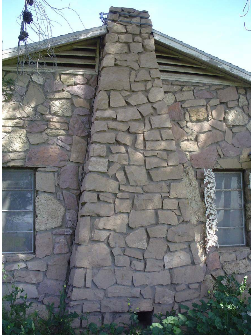
Original chimney on south façade of house showing different masonry pattern and gable vent detail, looking north.
