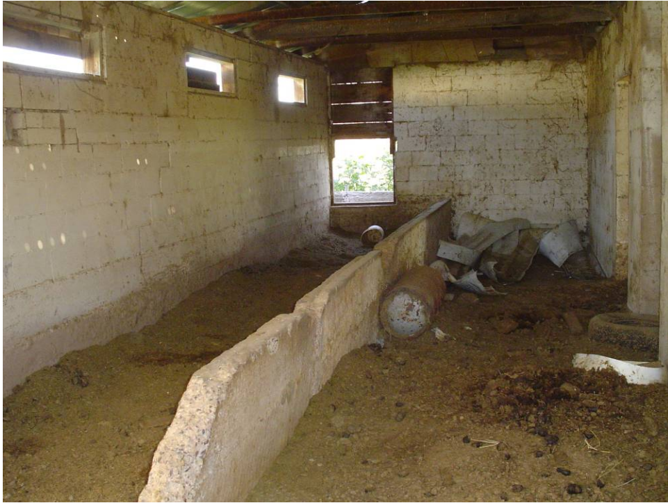
Interior west and north walls of west (milking) room, showing elevated cattle doorway and milking platform support wall with wear marks from cattle stanchion mounts, looking northwest.
