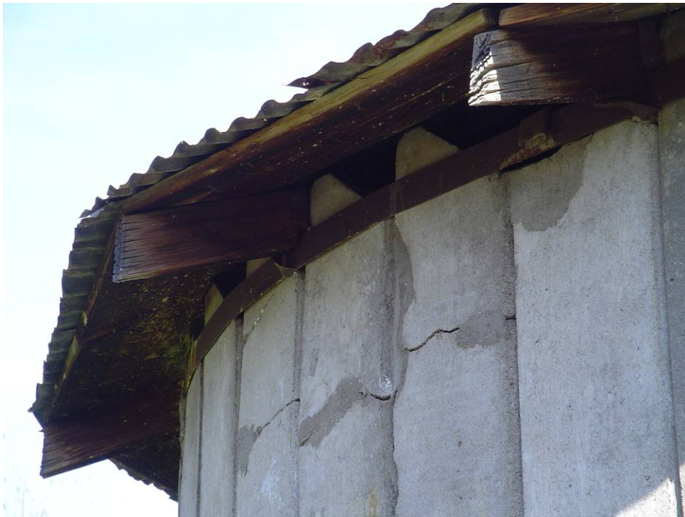
Detail of concrete stave silo wall/roof juncture.
