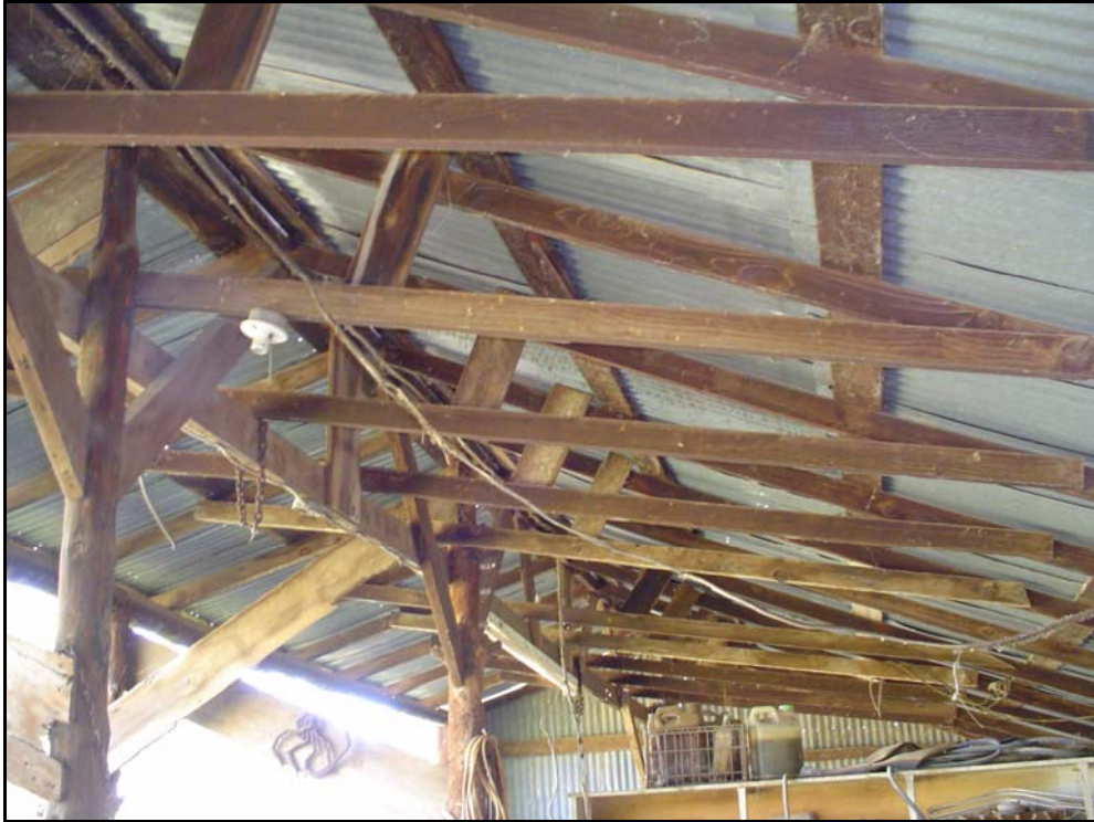
Figure 6.74. Hudson Farmstead: machine shop, interior truss system.
