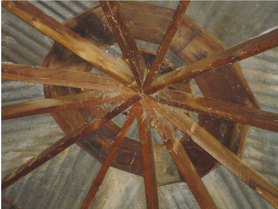
Interior roof structure of silo.
