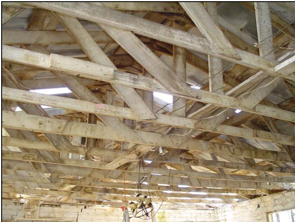
Figure 6.62. Hackin Farmstead: dairy flat barn, wood truss roof supports.
