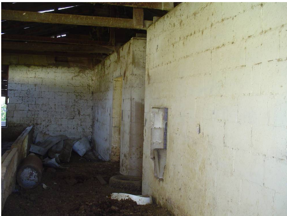
Interior west and north walls of west (milking) room, showing elevated cattle doorway and milking platform support wall with wear marks from cattle stanchion mounts, looking northwest.
