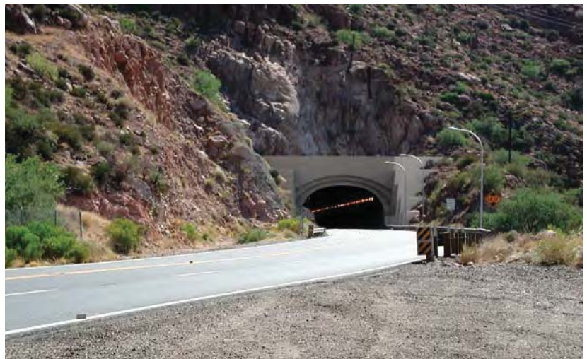
US 60 Queen Creek Tunnel: approximately 50' wide, carries 4-lanes of traffic, scarring to the ridge for the construction of the portal.
