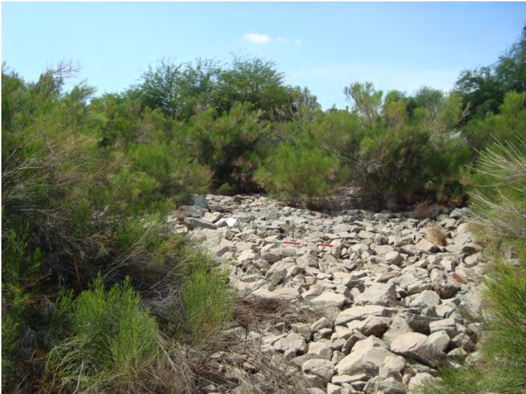
Photo 9. Constructed channel 3 (C3) facing northwest (upstream); rip-rapped segment; 4-foot-long scale
