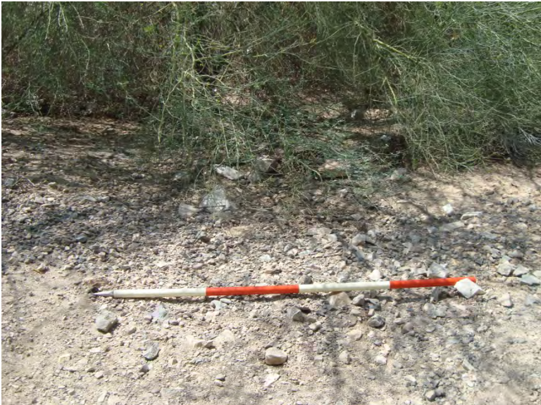
Photo 13. Constructed channel 4 (C4) facing northwest (upstream); 4-foot-long scale
