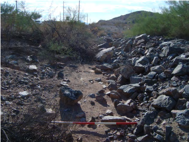
Photo 31. Stormwater drainage channel (S1) facing west (upstream); 4-foot-long scale
