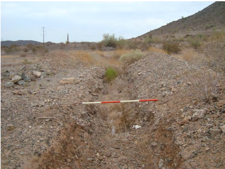
Photo 216. Constructed ditch (CD) facing northeast (upstream); 4-foot-long scale
