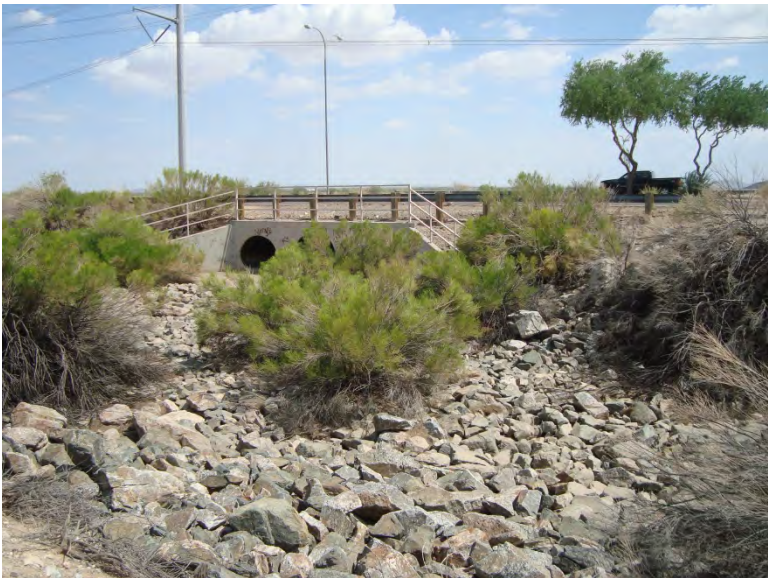
Photo 19. Constructed channel 4 (C4) facing southeast (downstream) toward Pecos Road
