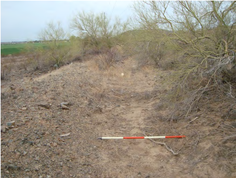
Photo 212. Constructed ditch (CD) facing north (upstream); 4-foot-long scale
