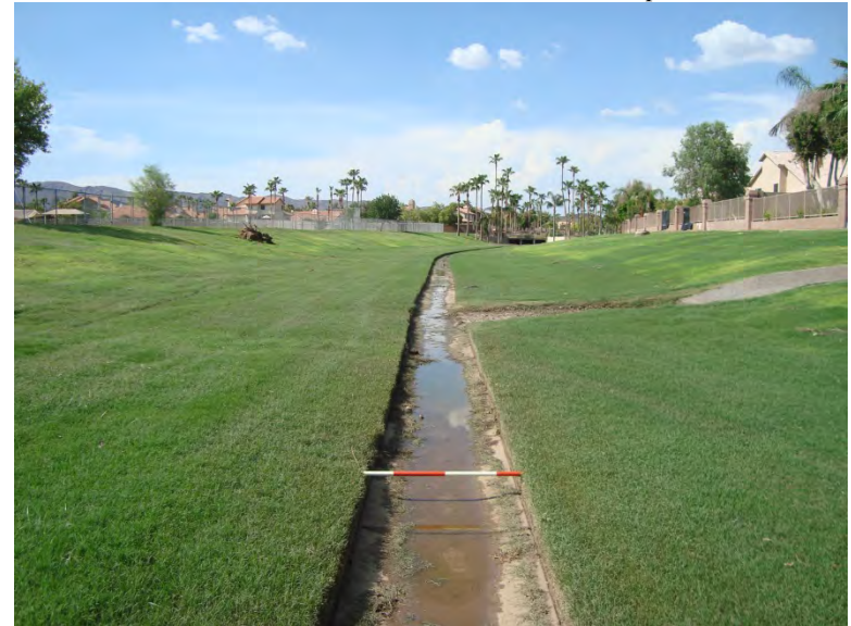
Photo 6. Constructed channel 1 (C1) facing north (upstream); OHWM at the break of slope; 4-foot-long scale
