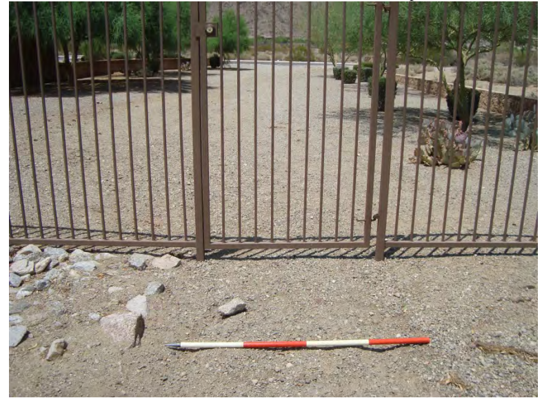
Photo 110. Stormwater feature (SF) conveying drainage from housing development facing north (upstream); 4-foot-long scale
