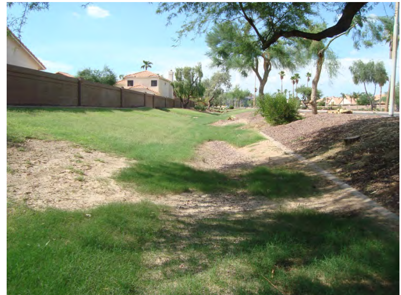
Photo 8. Constructed channel 2 (C2) along 32 nd Street facing north (upstream); provides stormwater drainage for development
