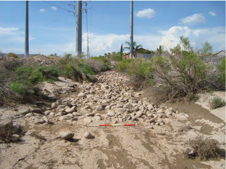
Photo 3. Wash 1 (W1) facing north (upstream); rip-rap lined channel near homes; 4-foot-long scale
