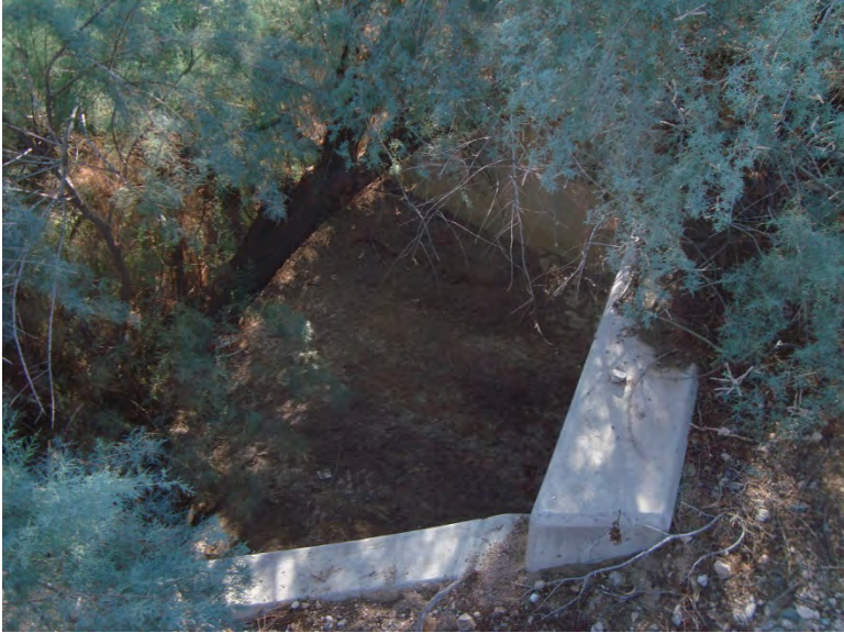
Photo 22. Wash 2 (W2) at culvert inlet
