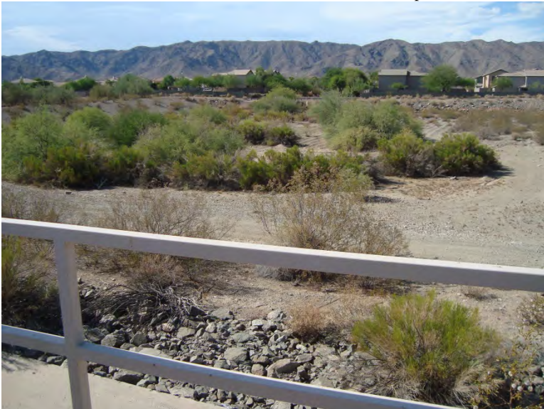
Photo 46. Detention basin (DB) near outlet facing northwest (upstream); no channel or OHWM to outlet
