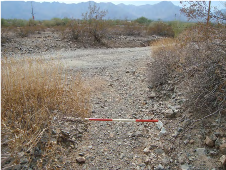
Photo 205. Wash 40 (W40) facing southwest (downstream); water crosses road and flows along road ditch; 4-foot-long scale
