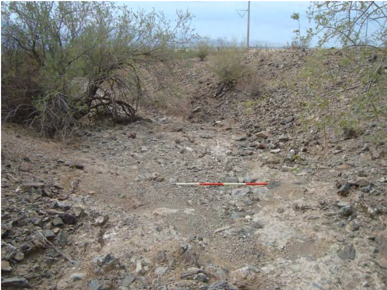
Photo 209. Wash 41 (W41) facing west (downstream); channel in area of bedrock; 4-foot-long scale
