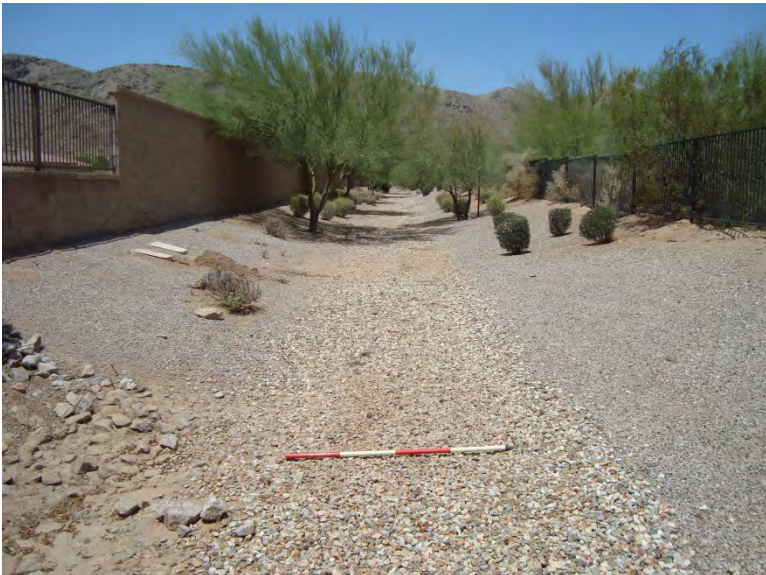
Photo 107. Constructed channel 7 (C7) facing north (upstream); 4-foot-long scale
