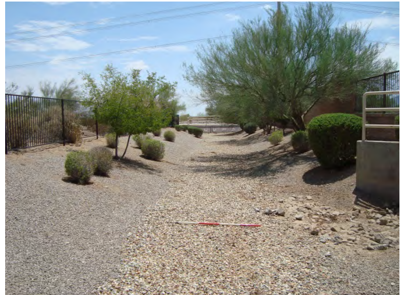
Photo 108. Constructed channel 7 (C7) facing south (downstream); 4-foot-long scale
