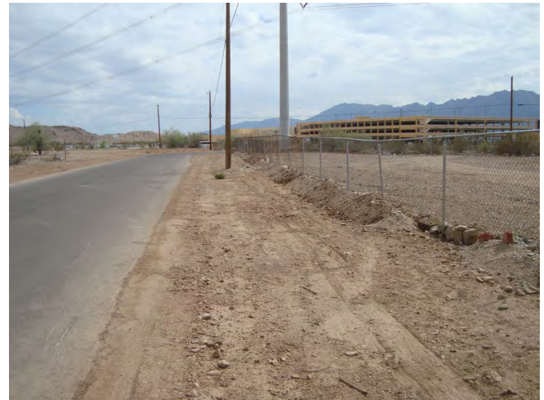
Photo 188. Wash 34 (W34) facing south (downstream); no channel; freshly graded road shoulder; water flows along edge of road
