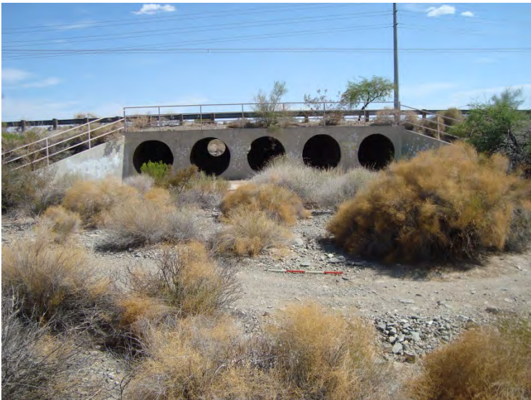
Photo 51. Constructed channel 6 (C6) facing south (downstream) to Pecos Road; 4-foot-long scale
