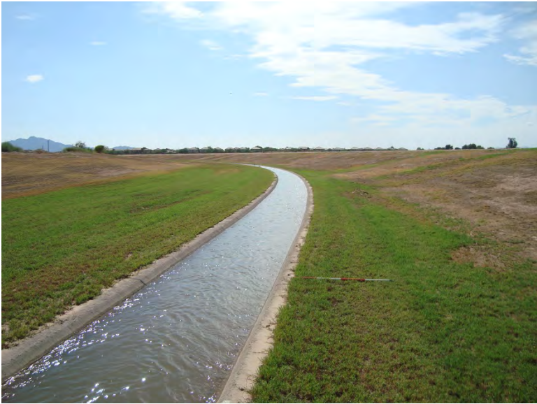
Photo 221. Laveen Conveyance Channel (LC) facing west (downstream); 4-foot-long scale
