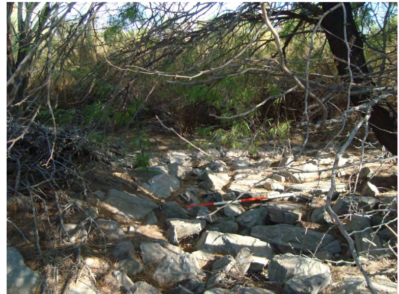
Photo 28. Constructed channel 5 (C5) facing southeast (downstream); rip-rapped; 4-foot-long scale
