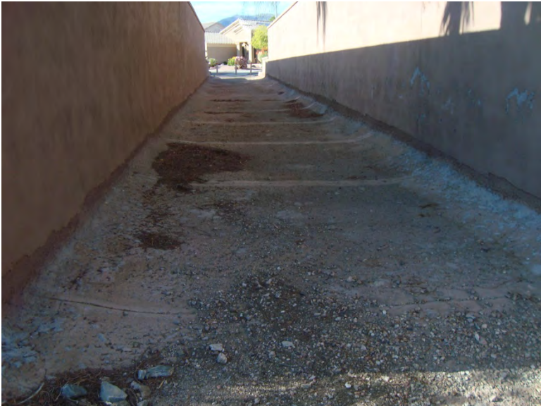
Photo 29. Stormwater drainage channel (S1) for development; facing north (upstream)
