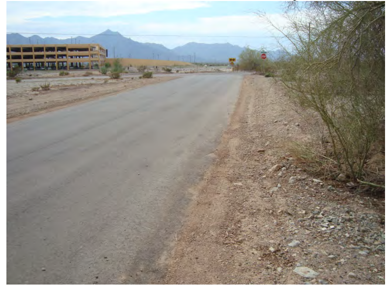
Photo 186. Wash 33 (W33) facing west (downstream) from outside survey boundary; no channel, water flows along edge of road
