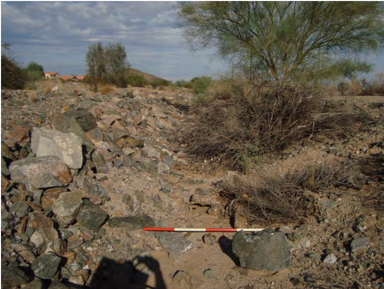
Photo 32. Stormwater drainage channel (S1) facing east (downstream); 4-foot-long scale
