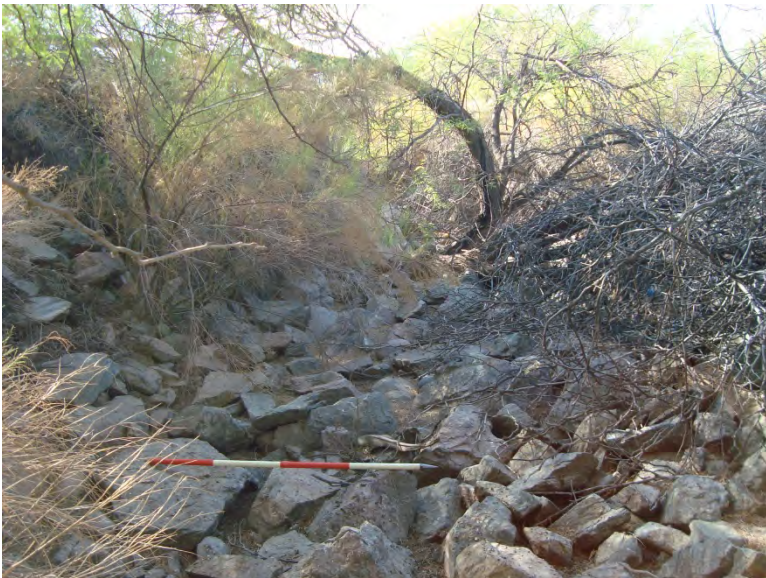
Photo 27. Constructed channel 5 (C5) facing northwest (upstream); rip-rapped; 4-foot-long scale
