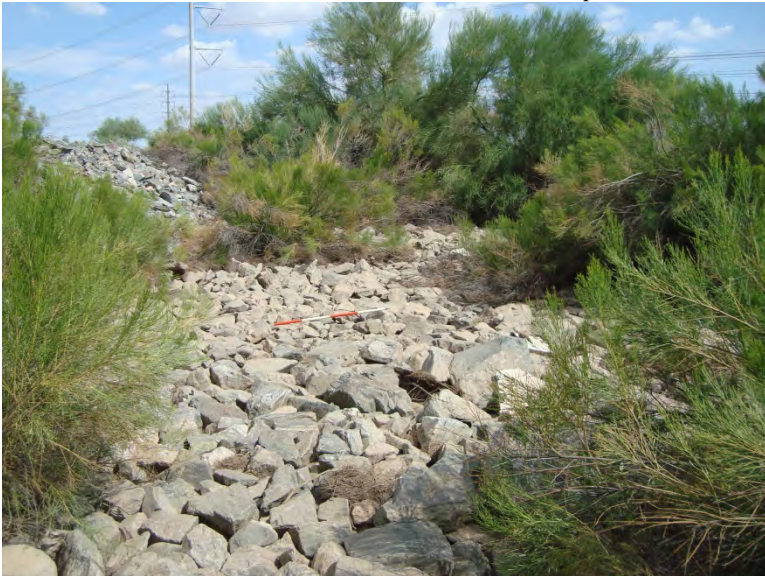
Photo 10. Constructed channel 3 (C3) facing southeast (downstream); rip-rapped segment; 4-foot-long scale
