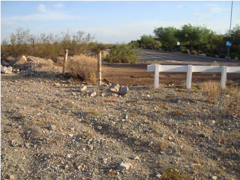
Photo 95. Wash 13 (W13) facing south (downstream); OHWM not visible but flow path could be seen in gravel; 4-foot-long scale
