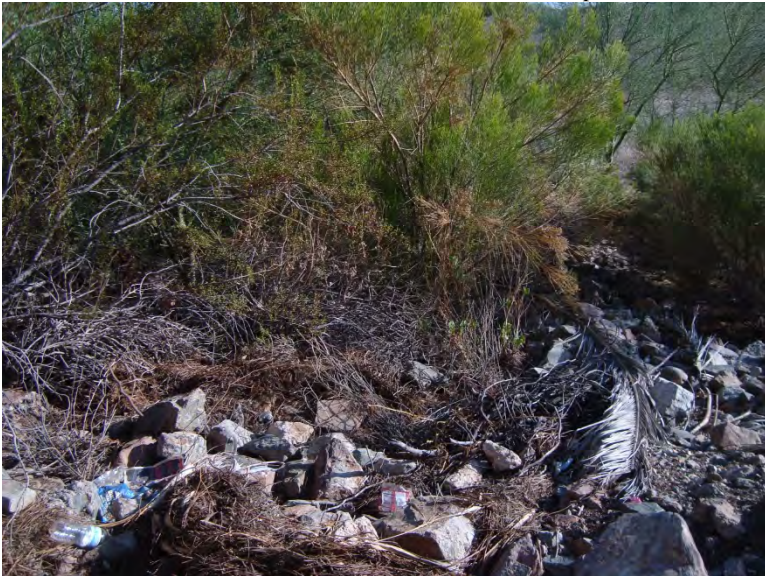
Photo 30. Stormwater drainage channel (S1) outlet; facing south (downstream)
