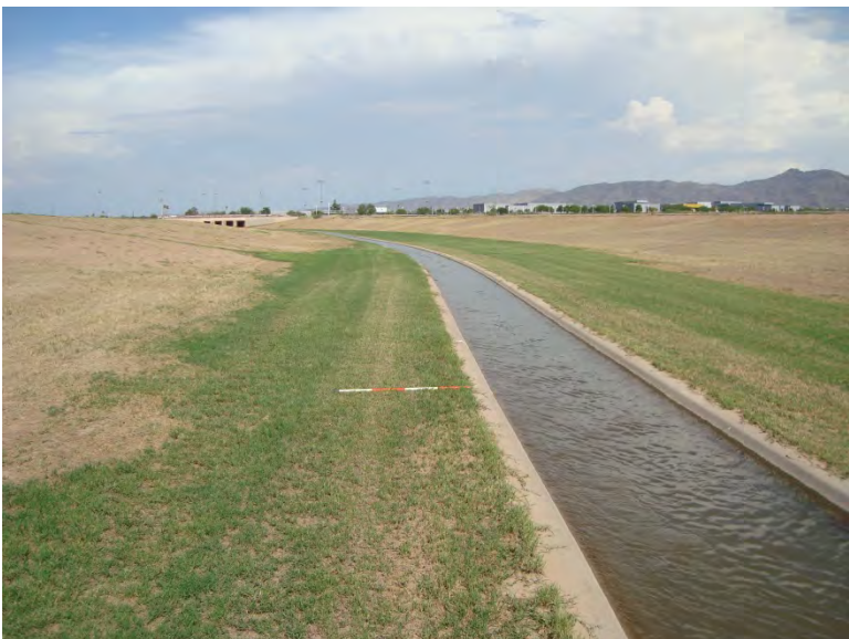
Photo 220. Laveen Conveyance Channel (LC) facing east (upstream); 4-foot-long scale
