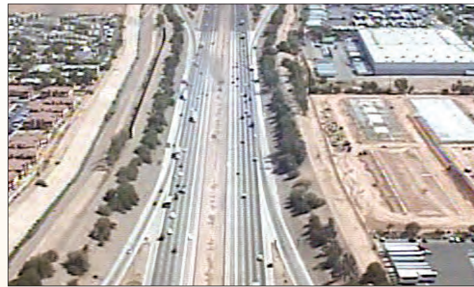
(b) I-10 at 71st Avenue, looking east
