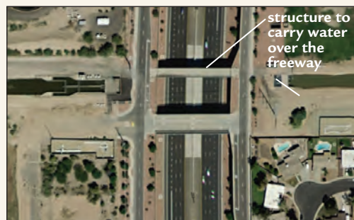
Channel over freeway
