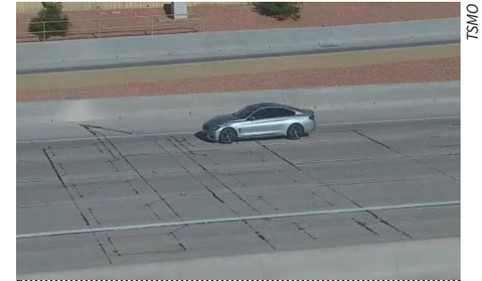
The black lines are the epoxy covering the saw cuts that house the loops, which detect the number of vehicles on the roadway.
