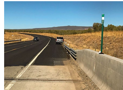
Before and after: Previously, bridge expansion joints had no snow plow markers, resulting in accidents, repair costs and delays in service.
