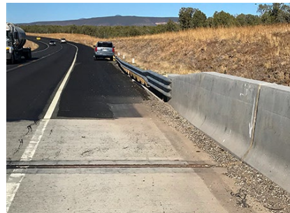
Before and after: Previously, bridge expansion joints had no snow plow markers, resulting in accidents, repair costs and delays in service.
