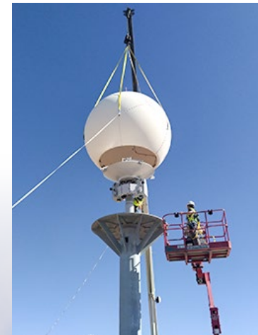
A long-range weather X-Band radar dish (pictured on left) is part of ADOT's Dust Detection and Warning System. It sits atop a 22-foot-tall pole at the State Route 87 interchange that can detect storms more than 40 miles away.
