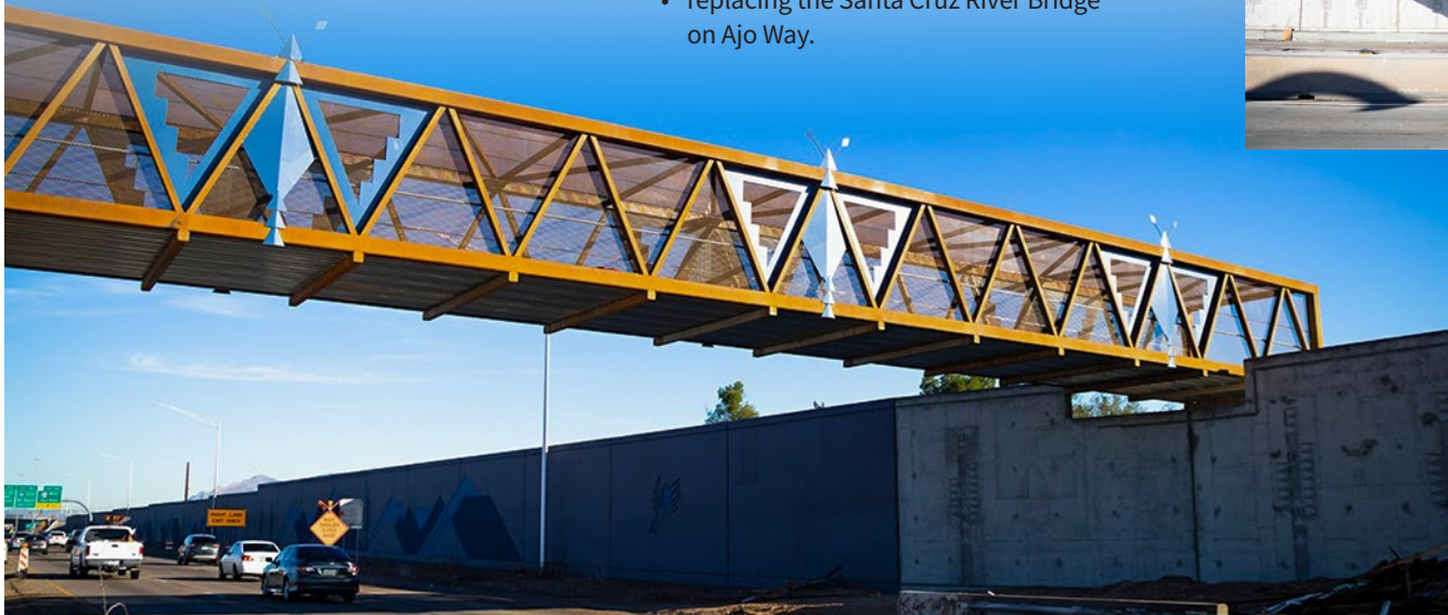
The new pedestrian bridge over Interstate 19 between Ajo Way and Irvington Road was installed in mid-January. It features ramps that are ADA compliant.
