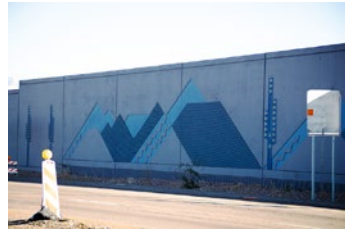
New sound walls along I-19 are part of the Phase 2 construction.
