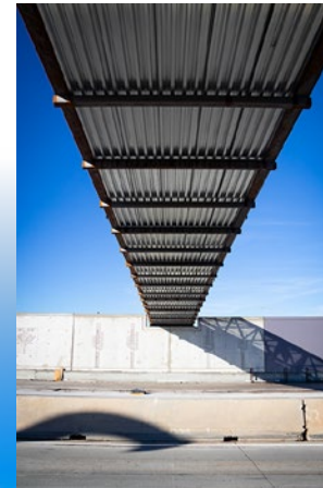
This is a view of the bridge from underneath.
