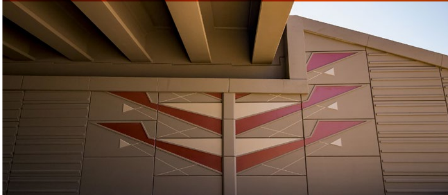
The Ocatillo Settlement pattern is on the abutment wall of the 40th Street bridge.
