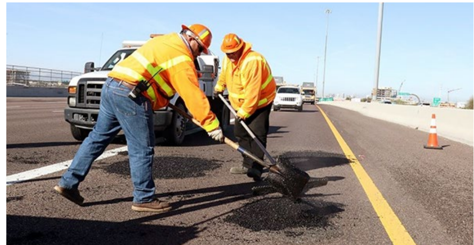
Workers repair potholes that resulted from the storm.
