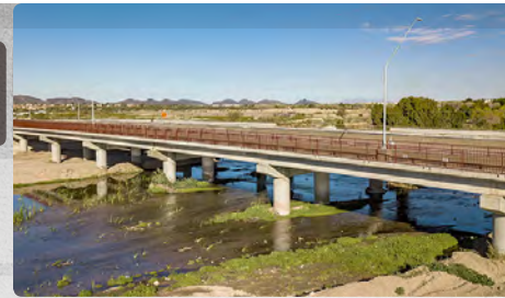
Ina Road is being widened to two lanes in each direction from I-10 west over new bridges crossing the Santa Cruz River.
