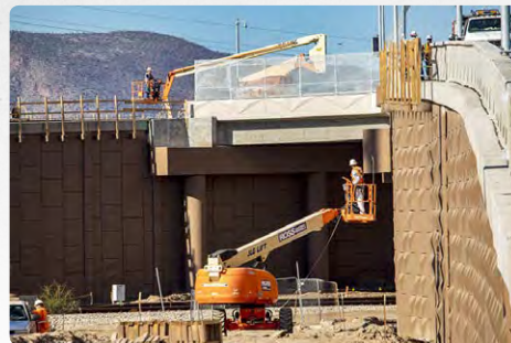
A new I-10 interchange at Ina Road is expected to be nearly completed by spring.
