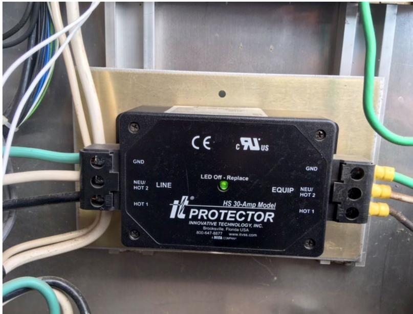
Surge suppression units installed on traffic signal cabinets protect equipment and prevent costly repairs.
