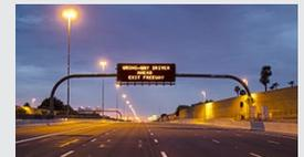
*This photo, taken by John Dougherty of ADOT Communications, shows a message alerting motorists that a wrong-way driver is ahead. Using thermal cameras, ADOT's wrong-way driver detection system alerts law enforcement when a vehicle enters the freeway traveling the wrong way. ADOT has received national awards for its first-in-the-nation system.*
