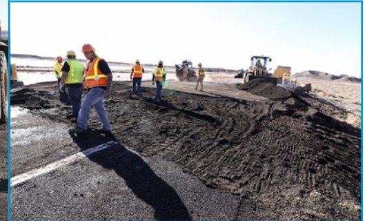
Crews used 500 cubic yards of material to restore US 89's base after floodwaters caused a 30-foot gap in this vital highway through northern Arizona.
