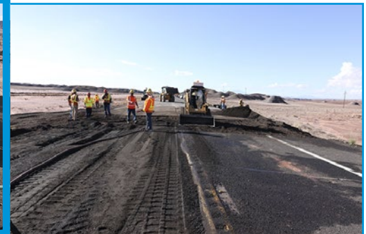
Crews applied 120 tons of asphalt pavement to repair US 89.
