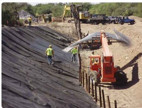
Crews place geotextile fabric during the emergency repair project last October.
