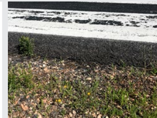
Pavement lip greater than 3-inches
