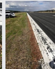
Pavement lip that has clean dirt to correct 3-inch lip
