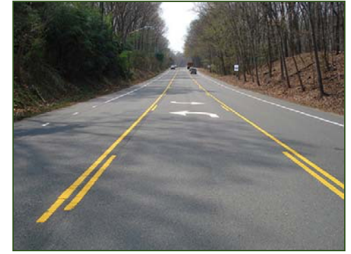
Photo Courtesy of FHWA
