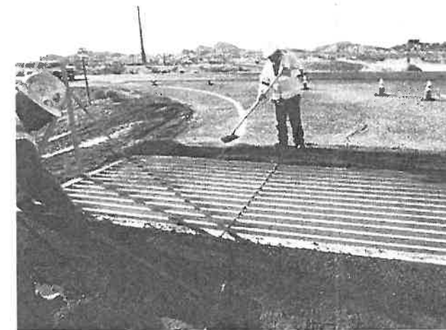
SR 95 Fencing Project - Cattle Guard Installation
