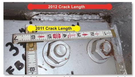
An example of where new cracks have grown in previous bridge inspection reports. While this was 6-years old, cracks found in 2017 now total nearly 100-ft in length, increasing 39% in one year from 2016! Even repaired cracks are cracking again!
