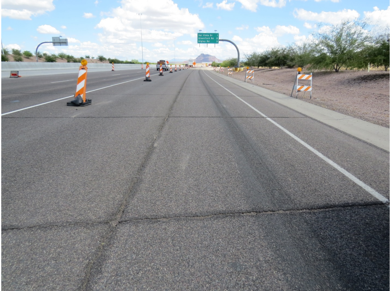
Cracking (Unacceptable)
