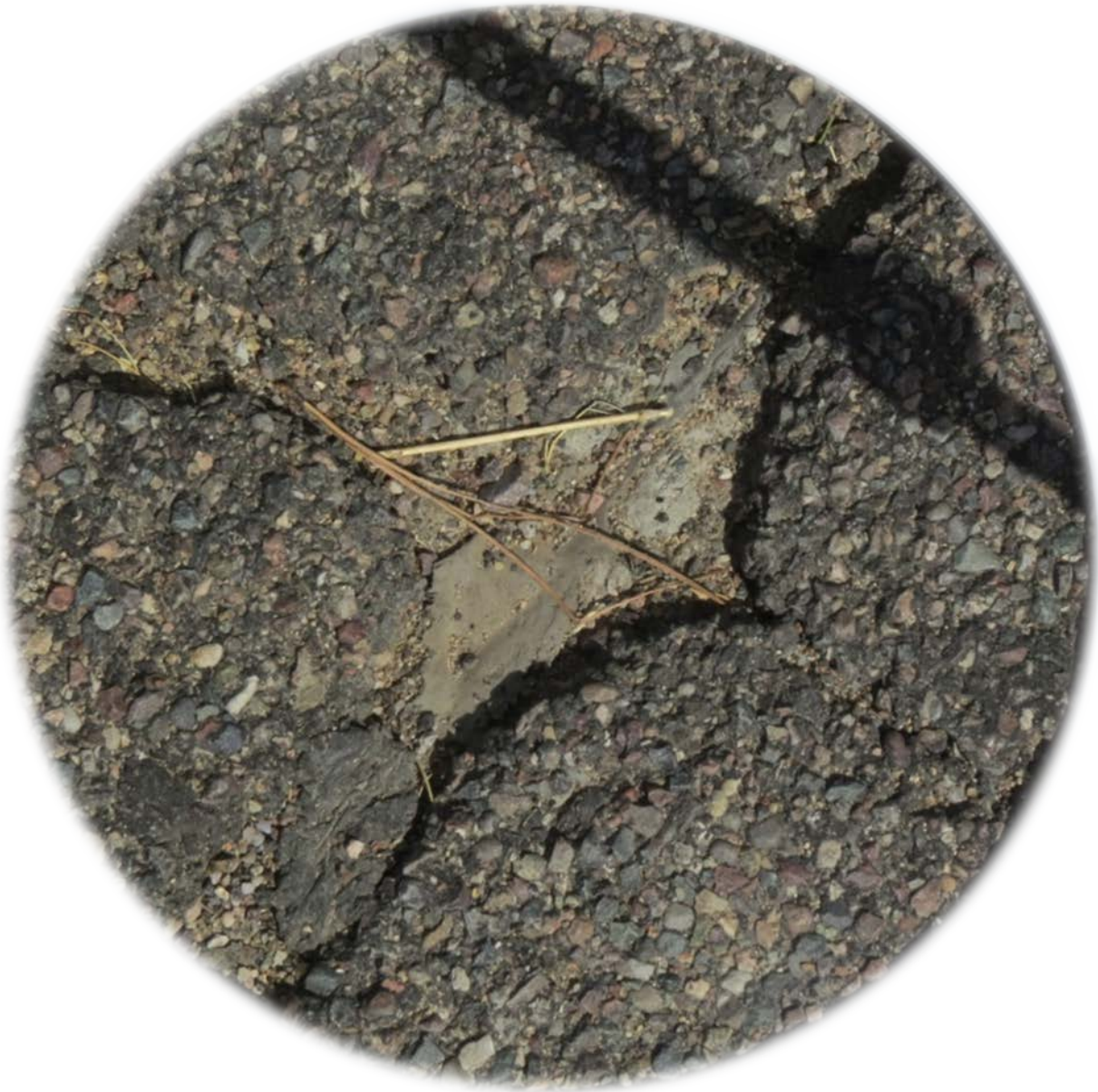
Delamination (Unacceptable)
