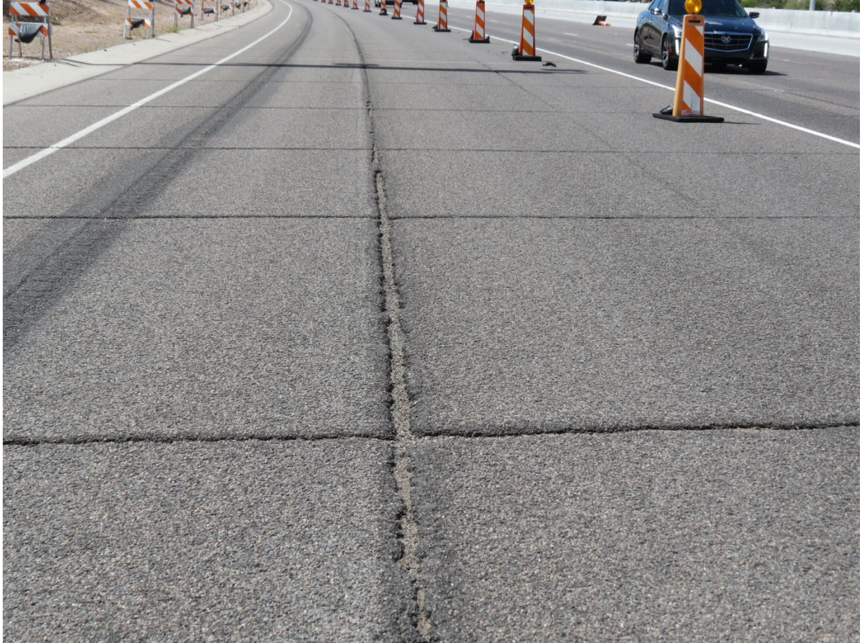
Cracking (Unacceptable)
