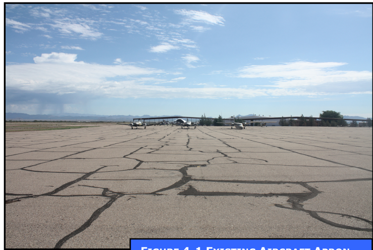
FIGURE 4-1 EXISTING AIRCRAFT APRON
