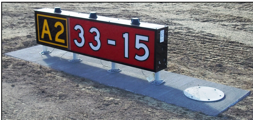
FIGURE 3-5 TYPICAL HOLDING POSITION SIGN
