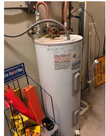
Figure 8: 30 gal DHW Storage Tank
