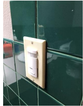
Figure 3: Occupancy Sensor in the Restroom
