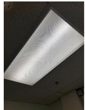
Figure 1: Fluorescent Lighting Fixtures in the ATCT
