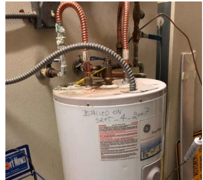
Figure 7: Uninsulated copper DHW pipes
