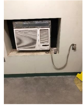
Figure 6: Window Unit in ATCT
