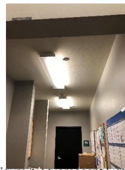
Figure 1: Fluorescent Lighting Fixtures in the Hallways
