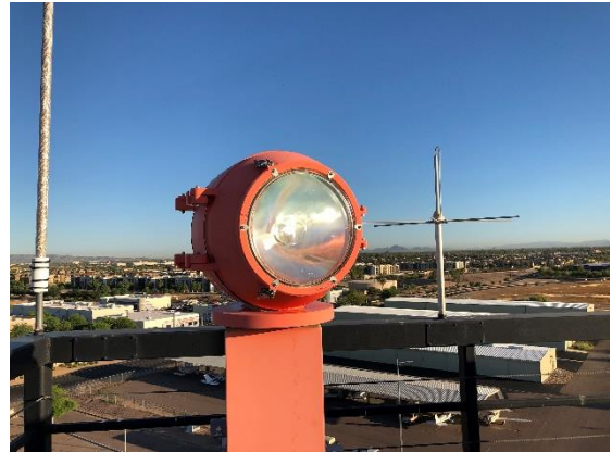
Figure 3: Beacon Light at top of ATCT
