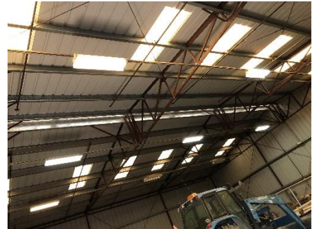
Figure 2: Linear Fluorescent Fixtures in the Maintenance Building
