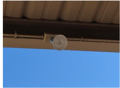
Figure 2: Existing Canopy Lighting Fixtures
