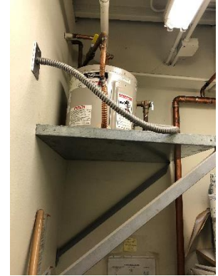
Figure 7: 6 Gallon DHW Storage Tank
