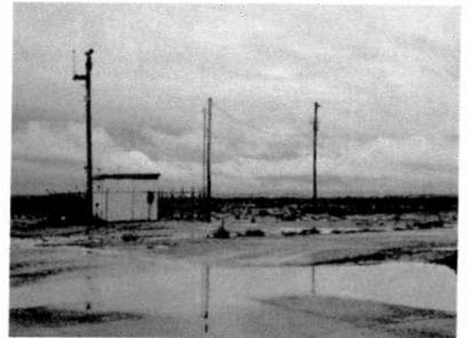
AIRPORT BEACON (NOTE APRON DRAINAGE)
