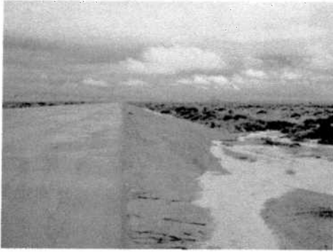
RUNWAY PAVEMENT AND SAFETY AREA
