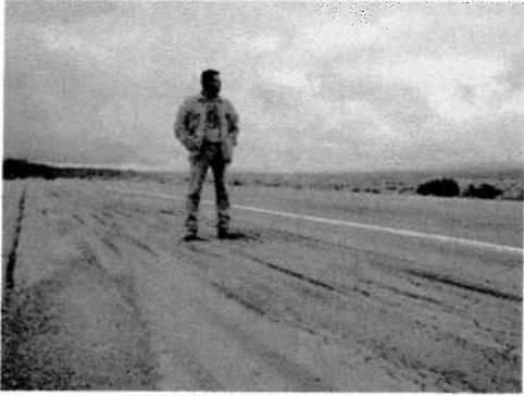
RUNWAY PAVEMENT (NOTE RUTTING)
