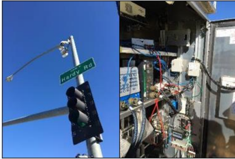
Figure 7. Pole-Mounted Communications and Interior of Traffic Cabinet at Intersection of SR 77 and Hardy Road (September 15, 2016)
