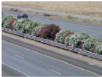
Figure 2. Thrie Beam Barrier
