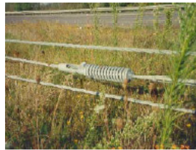
Figure 3. Three-Cable Barrier 7
