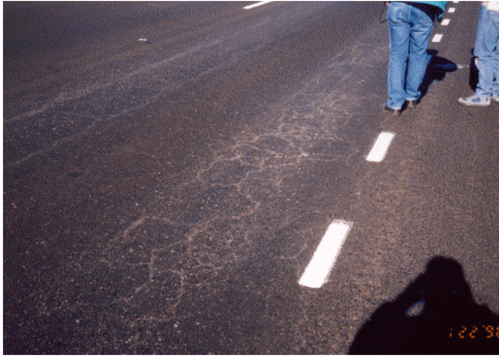
Photo No. 1 Fatigue Cracking in 1" Superpave Section (04A902)
