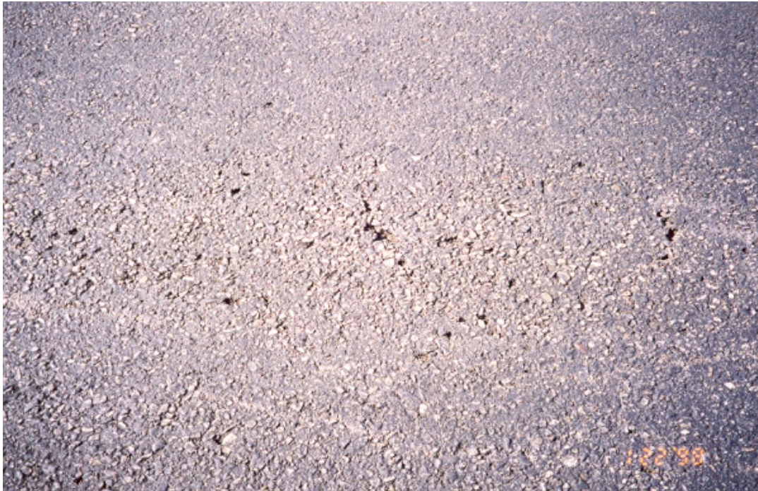
Photo No. 5 Segregation Evident in Superpave Sections
