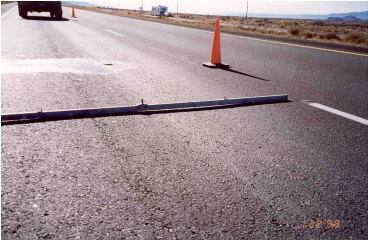
Photo No. 2 Rutting on 3/4" Superpave Section (040902)
