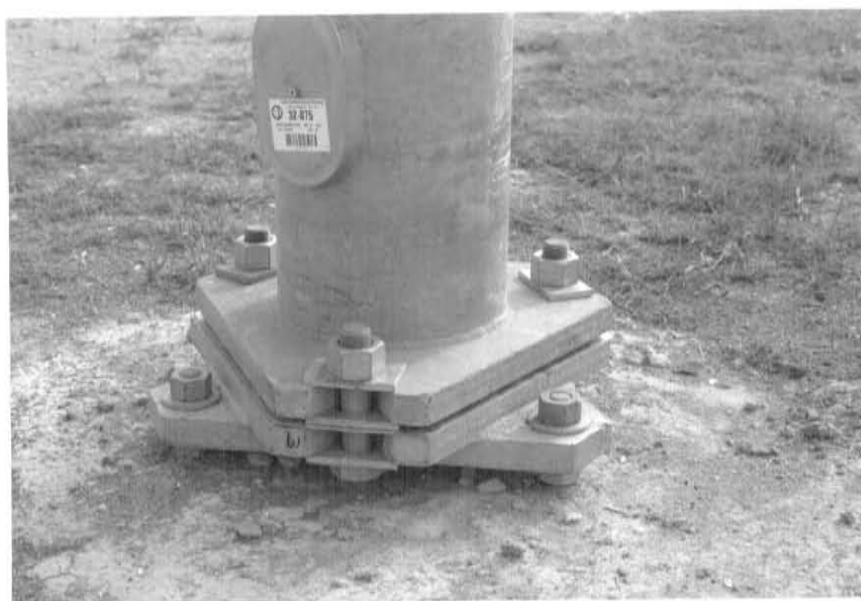
Figure 29. 12.2-m (40-ft) Arizona slip-away base luminaire support.
