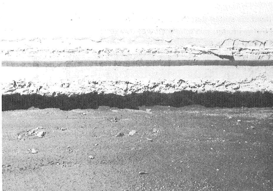
Figure 17 - Erosion Beneath PCC Pavement
