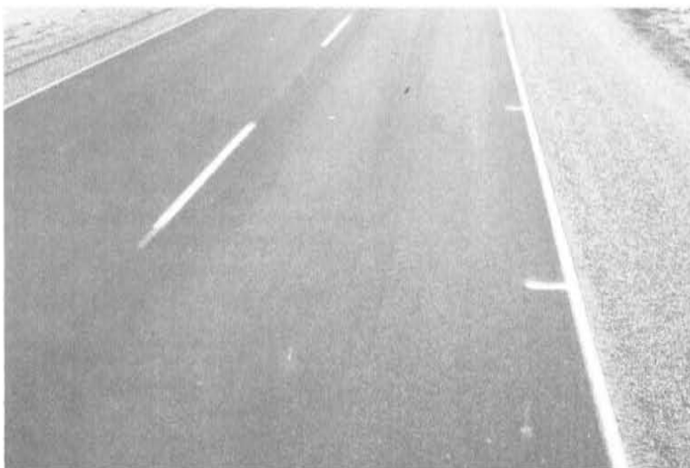
Figure 12. Typical Photo History of Cracking, Asphalt Rubber Between AC Overlay and ACFC, T.S. #3, Sta 317+75-318
