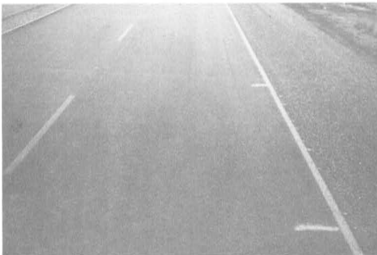
Feb. 6, 1973 0% Cracking After Overlay
