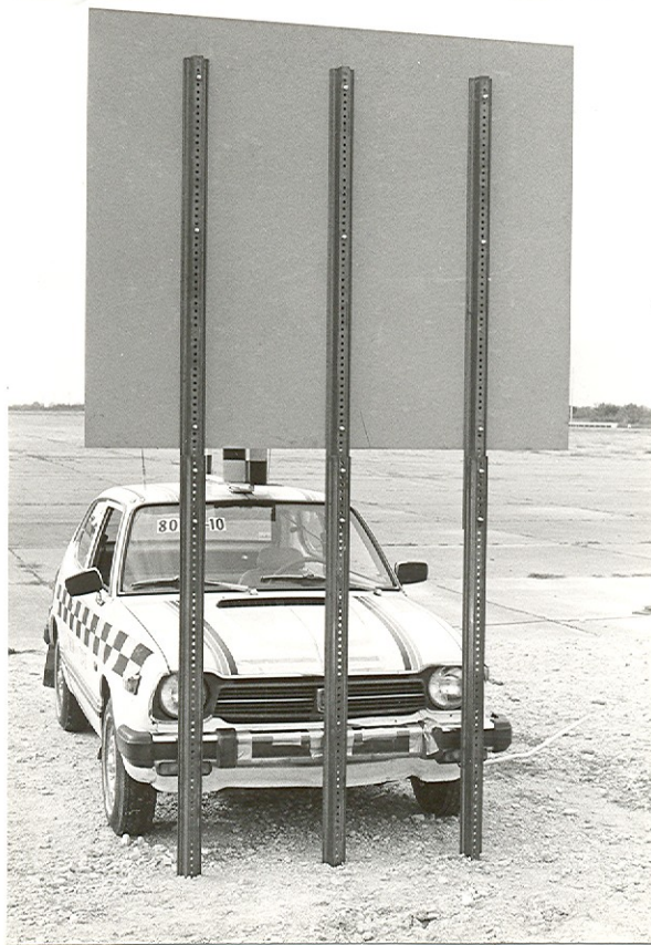
FIGURE A-78. RELATIVE POSITIONS OF TEST VEHICLE AND SIGN INSTALLATION FOR TEST 10.
