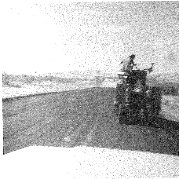
FIGURE 9: SURFACE COMPACTION, SPRAY-ON APPLICATION
