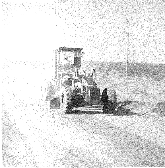
FIGURE 7: ROAD SURFACE PREPARATION, SPRAY-ON APPLICATION
