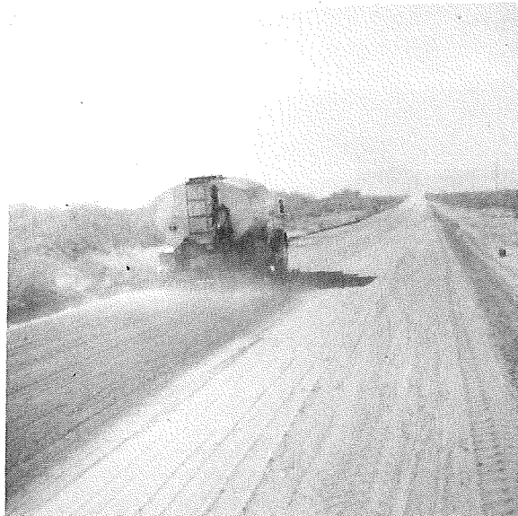
FIGURE 8: CHEMICAL SPRAY-ON APPLICATION
