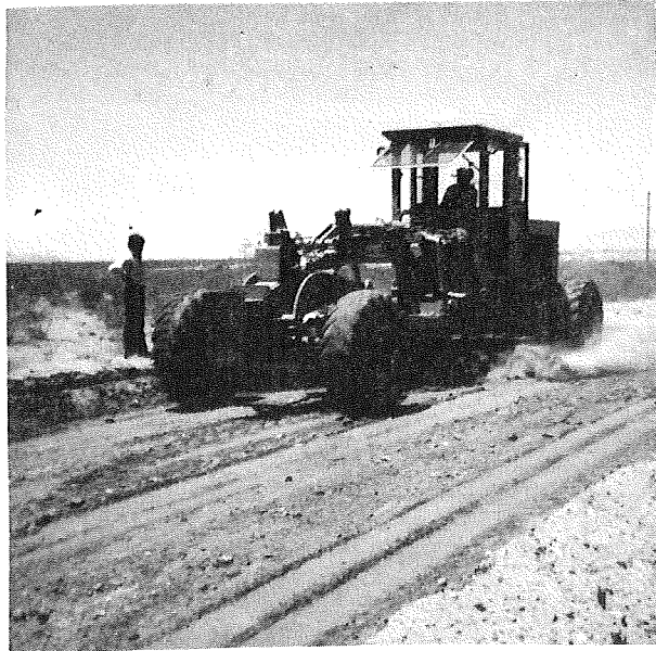
FIGURE 12: BLADE-MIXING OF SURFACE SOIL
