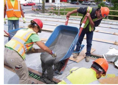
Figure 1. (a) The first UHPC bridge constructed in the U.S (in Wapello County, IA), (b) casting of longitudinal connections between deck-bulb-tee girders (Route 31 Bridge, Lyons, NY). Both figures courtesy of FHWA ( https://www.fhwa.dot.gov/publications/research/infrastructure/structures/11038/ )
