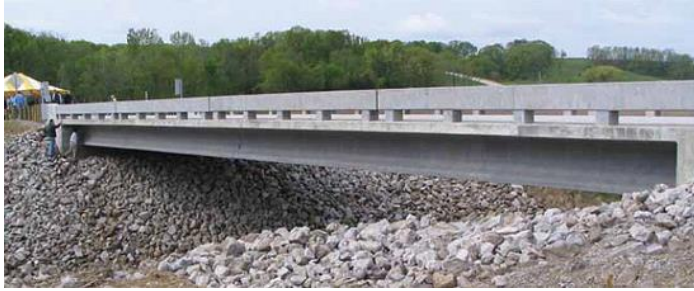
Figure 1. (a) The first UHPC bridge constructed in the U.S (in Wapello County, IA), (b) casting of longitudinal connections between deck-bulb-tee girders (Route 31 Bridge, Lyons, NY). Both figures courtesy of FHWA ( https://www.fhwa.dot.gov/publications/research/infrastructure/structures/11038/ )
