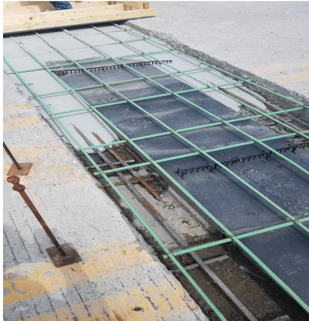
Figure 138. Transverse (LLC) joints filled with UHPC
