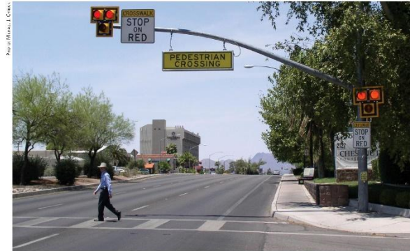
Example of a HAWK treatment in Tucson, Arizona. [Note: The pedestrian is Richard Nassi, developer of the HAWK.]
