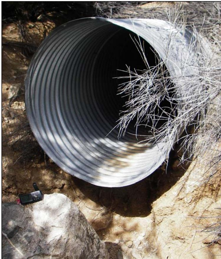
**Figure 11. Example of a Perched Entrance to a Drainage Culvert Running Underneath US 93.**
