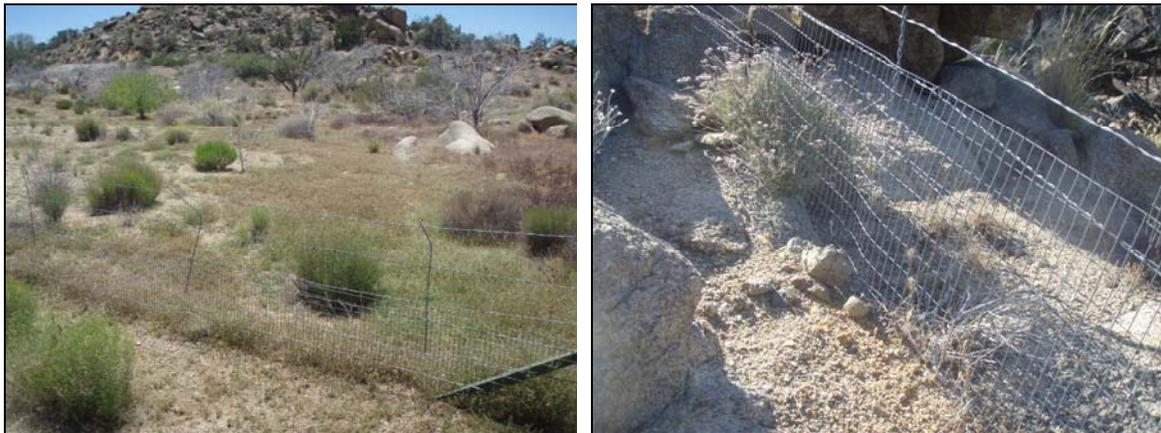
**Figure 5. Examples of Desert Tortoise Exclusion Fencing Installed during the US 93 Boulders Reconstruction Project.**
