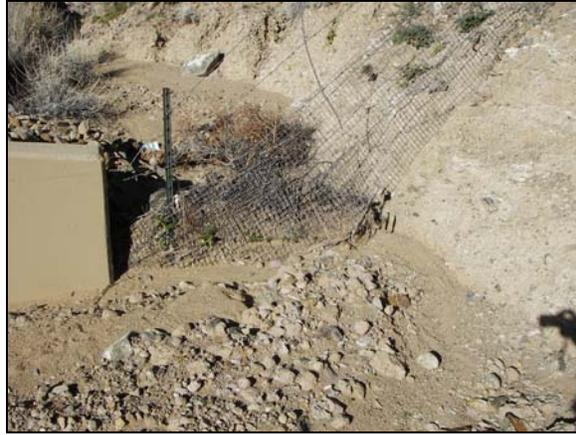
**Figure 38. Example of Erosion Damage to Connection between Fencing and Culvert Wing Wall.**
