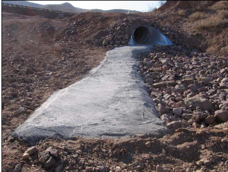
**Figure 43. Desert Tortoise Path Installed along US 93 near the Hoover Dam.**
