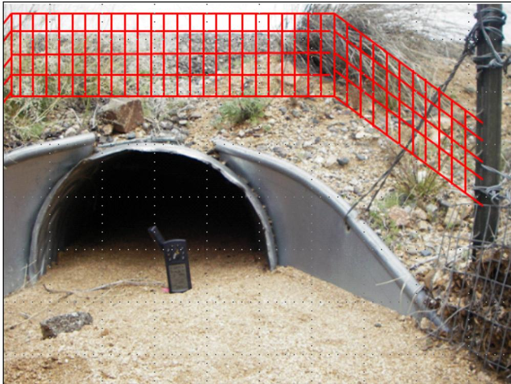
**Figure 39. Example of Alternative Fencing Placement Where Hydrology and Topography Are Likely to Damage Fencing (see Figure 38).**
