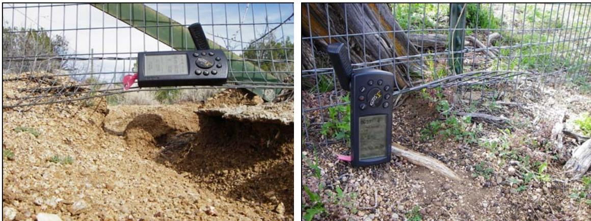
**Figure 10. Examples of a Structural Fencing Breach (Left) Caused by Erosion and Biological Breach (Right) Caused by Animals Pushing through a Nonburied Fencing Segment.**
