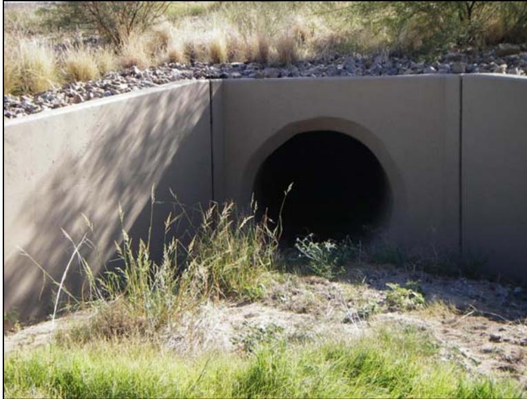
**Figure 9. Underpass Structure Designed to Facilitate Desert Tortoise Movement within the US 93 Project Area.**
