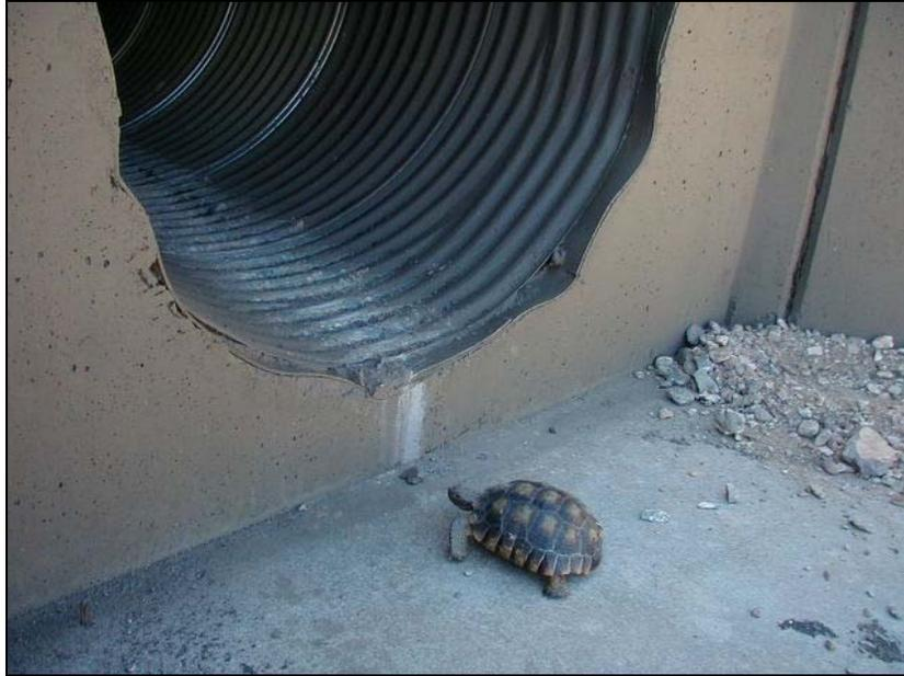
**Figure 42. Tortoise Use of Underpass Structure Inhibited by Perched Culvert Entrance.**
