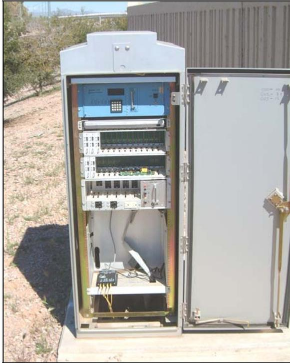
**Figure 2: FMS Cabinet with Inductive Loop Equipment**
