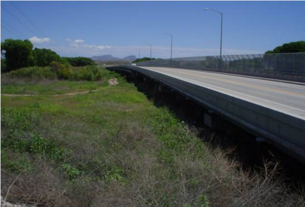
Figure 10. The 40-Foot-Wide Mitigation Strip Along the West Side of the SR 75, Gila River Bridge #311 Project Site.
