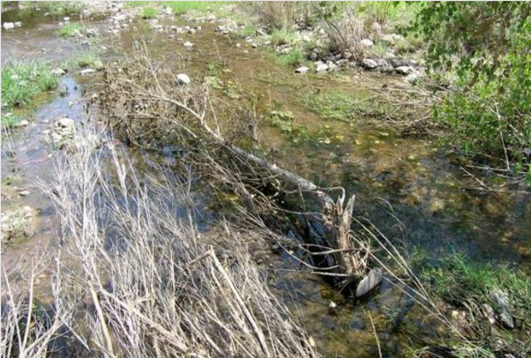
Figure 12. Pole Planting Knocked Down by Flooding at Peck Canyon Bridges Project Site, Between the Frontage Road and the I-19 Bridges.
