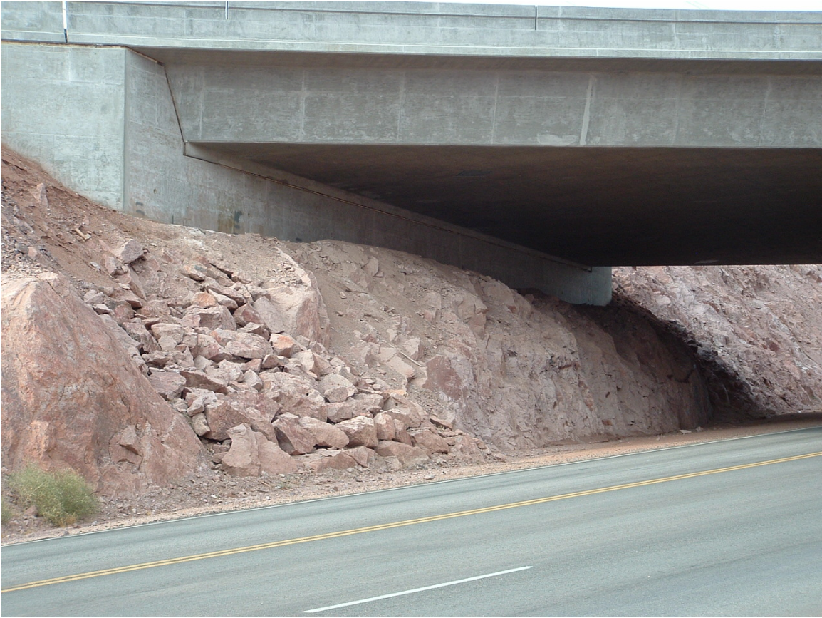
Appendix 11. Shelf below abutment at an underpass, Highway 93, Nevada
