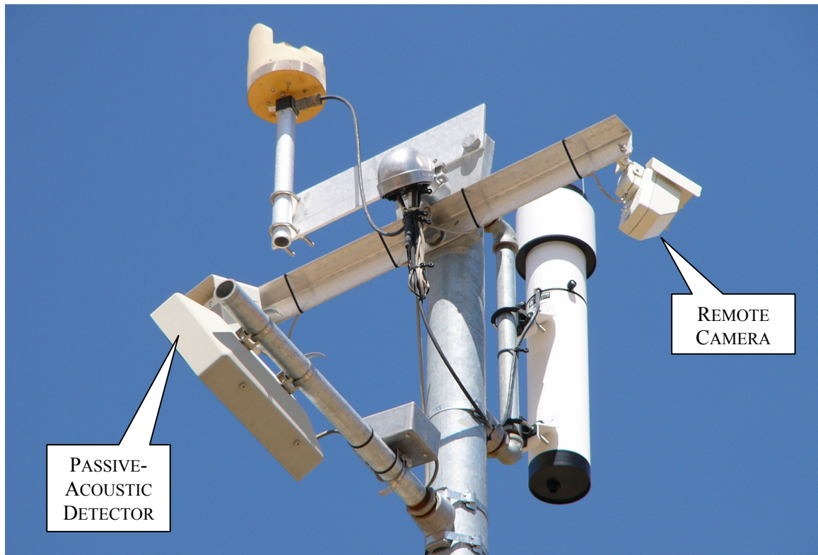
Figure 5: RWIS Sensor Assembly
