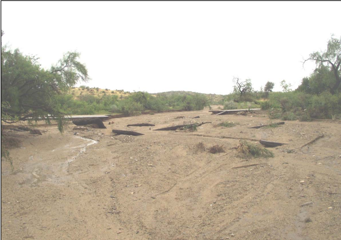
Figure 13 – Road Wash-Out on SR 186
