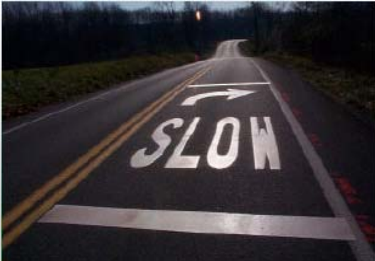
Figure 5.7: Advanced Curve Warning Markings Source: Bryer 2000
