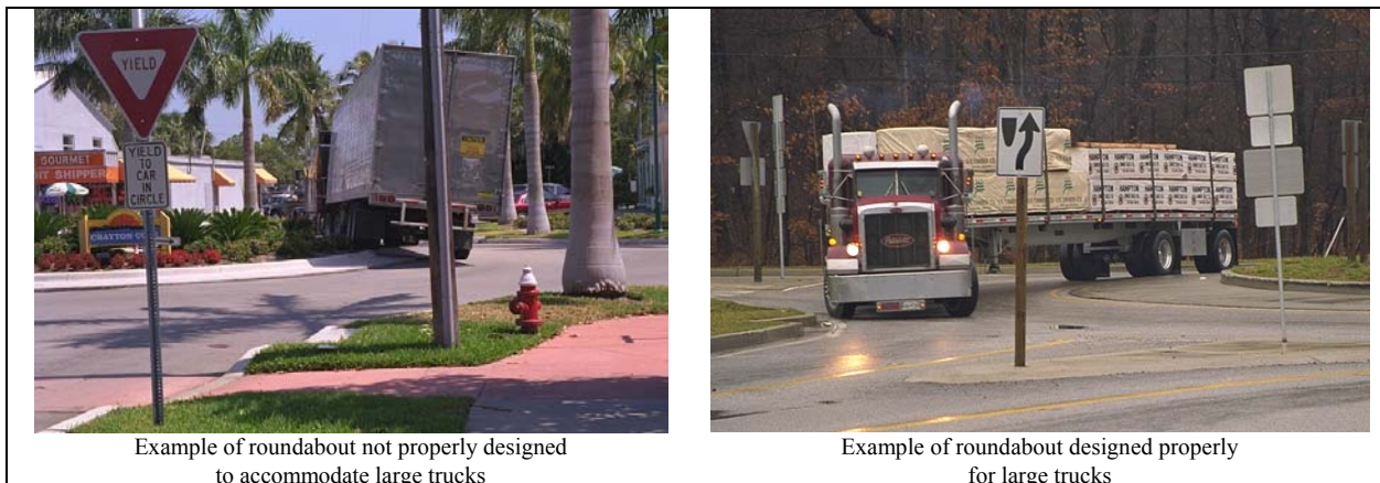
Figure 60 Truck Accommodations at Roundabouts
