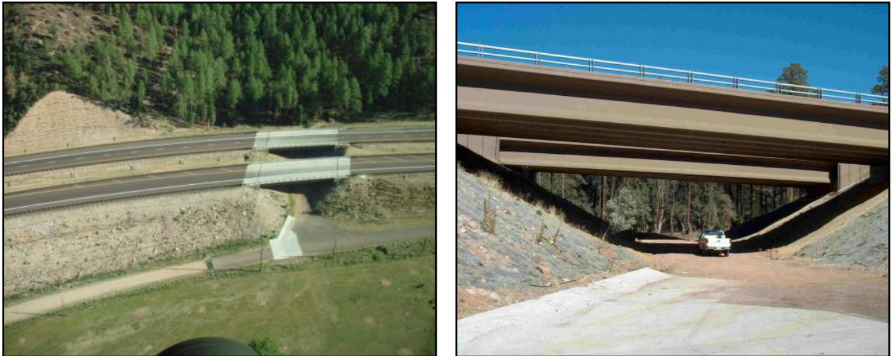
Figure 11.2. Aerial (left) and entry (right) views of the East Little Green Valley underpass looking north. Note how the underpass connects ponderosa pine forest to the meadow complex at Little Green Valley (left) and the 2:1 sloped earthen sides (right).
