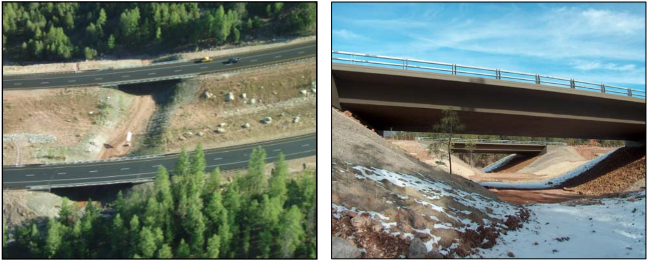
Figure 11.3. Aerial (left) and entry (right) views of the Pedestrian-Wildlife underpass looking north. Note how the underpass connects ponderosa pine forest on both sides of the highway and its wide atrium between bridges (left), and the high visibility through the underpass from the approaches (right).
