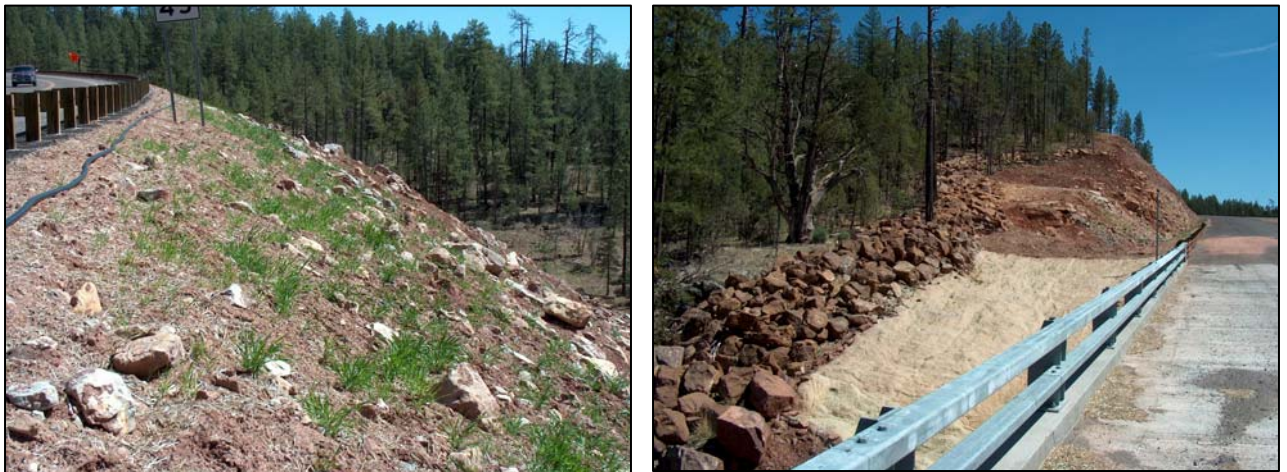
Figure 7.2. Alternatives to fencing to deter at-grade wildlife crossings along the Christopher Creek section of State Route 260, Arizona. The steep 4:1 fill slopes below guard rails (left), boulder rip-rap (“elk-rock”) and steep cut slopes (right) were evaluated as alternative treatments to fencing.
