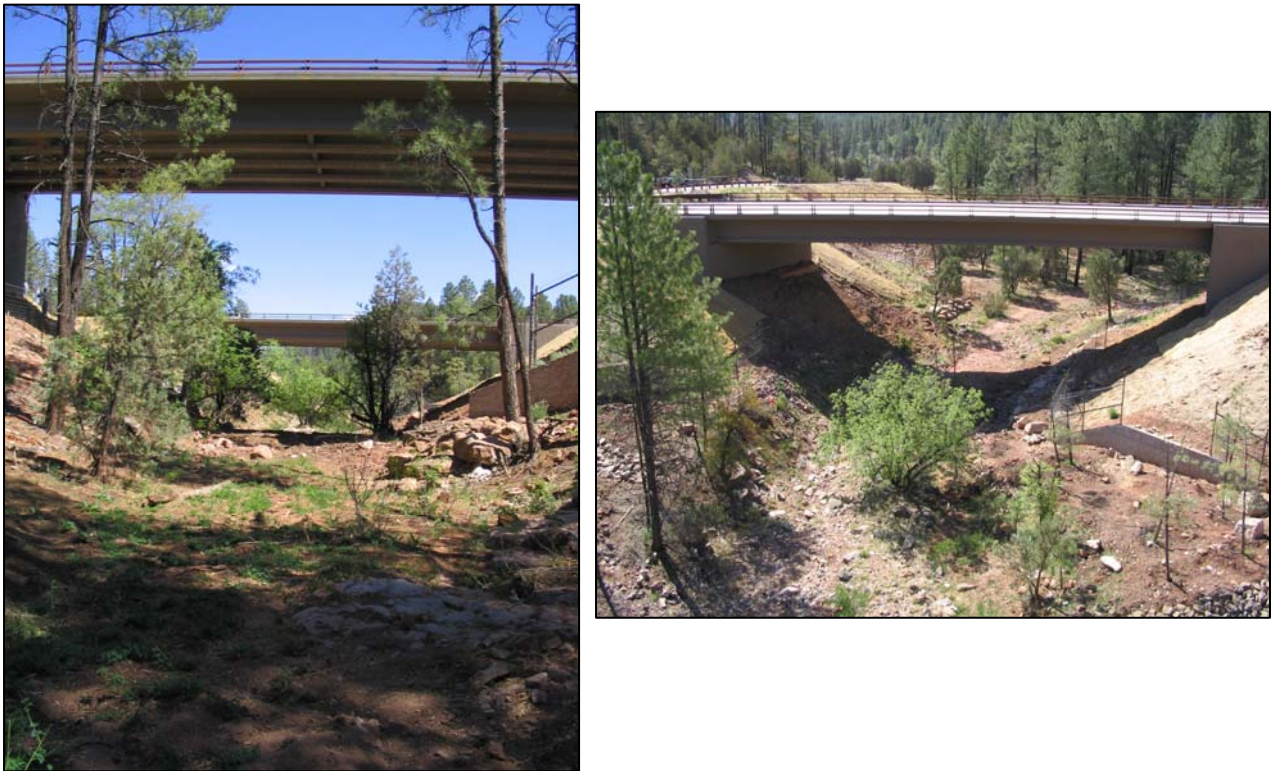
Figure 4.6. Indian Gardens wildlife underpass on the Kohl's Ranch section of State Route 260, Arizona, completed in March 2006. The design of this underpass was modified to eliminate concrete walls below the bridge spans for soil stabilization thus opening up the floor of the underpass (left) and preserving natural vegetation. The right photo was taken from the eastbound lanes bridge looking north toward the westbound lanes bridge. Note the escape ramp in the lower right hand portion of the right photo.
