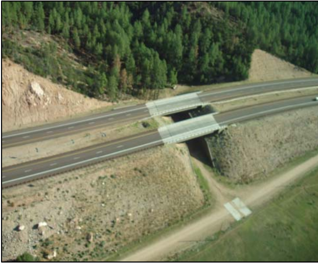
Figure 11.1. Aerial (left) and entry (right) views of the West Little Green Valley underpass looking north. Note how the underpass connects ponderosa pine forest to the meadow complex at Little Green Valley (left) and the concrete mechanically stabilized earth (MSE) walls (right).
