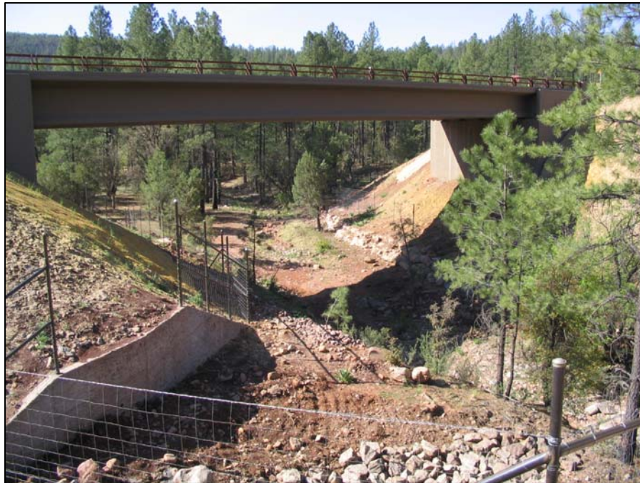
Figure 11.10. The Indian Gardens wildlife underpass on the Kohl's Ranch section (looking north from the east-bound lanes bridge), State Route 260, Arizona, where nearly all originally-planned concrete walls were removed upon construction, widening the underpass floor for wildlife passage, retaining native vegetation, and improving openness. The wall on the lower left corner of the photo is associated with a wildlife escape ramp (note the gap in the fencing).
