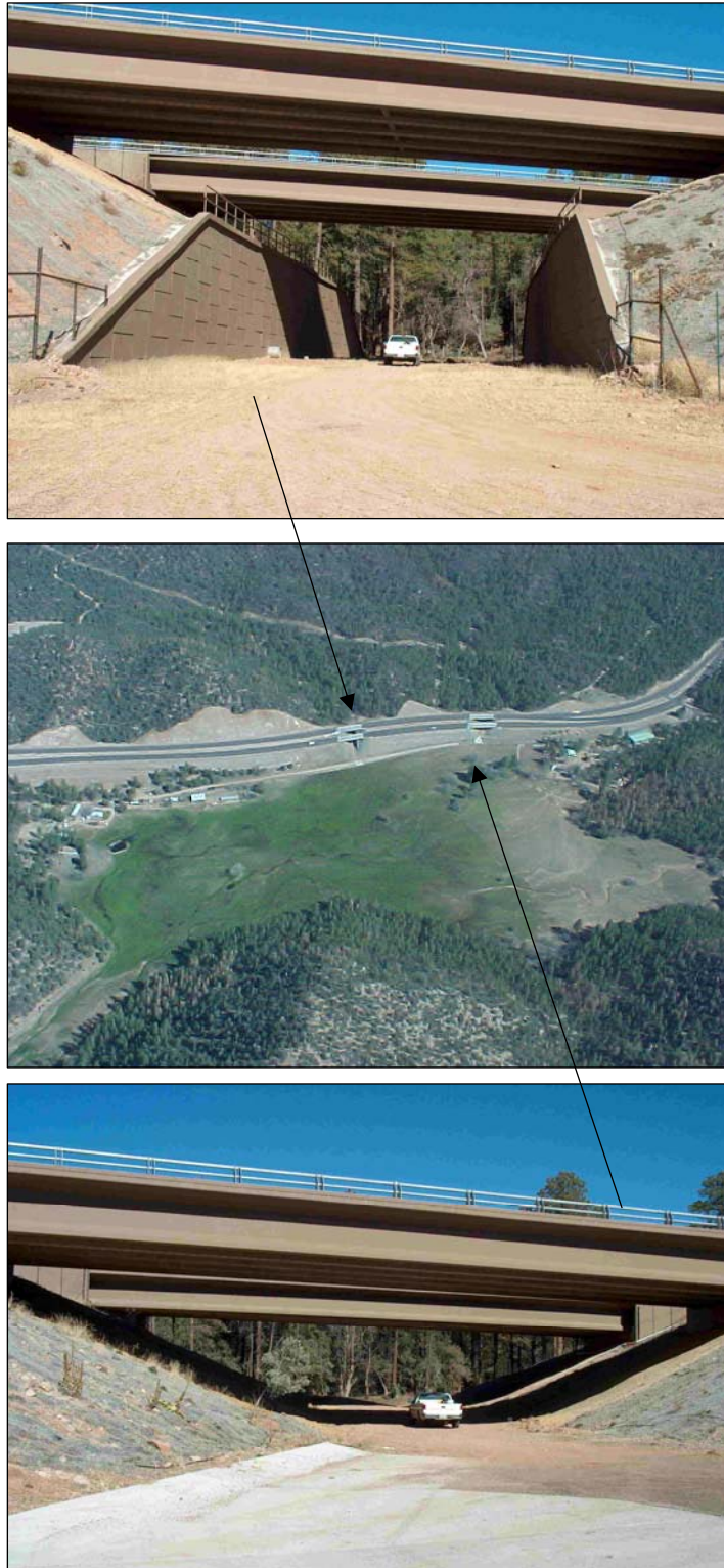
Figure 4.1. Little Green Valley riparian-meadow complex (center photo) adjacent to State Route 260 in Arizona, into which the west (top photo) and east (bottom photo) wildlife underpasses open. Note their proximity and the different soil stabilization features, the west with concrete walls, and the east with 2:1 sloped earthen sides.
