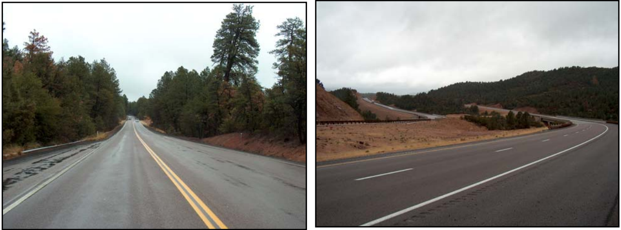
Figure 3.2. The existing narrow two-lane roadway (left; Doubtful Canyon section) is being reconstructed to a four-lane divided highway (right; Preacher Canyon section), State Route 260, Arizona.
