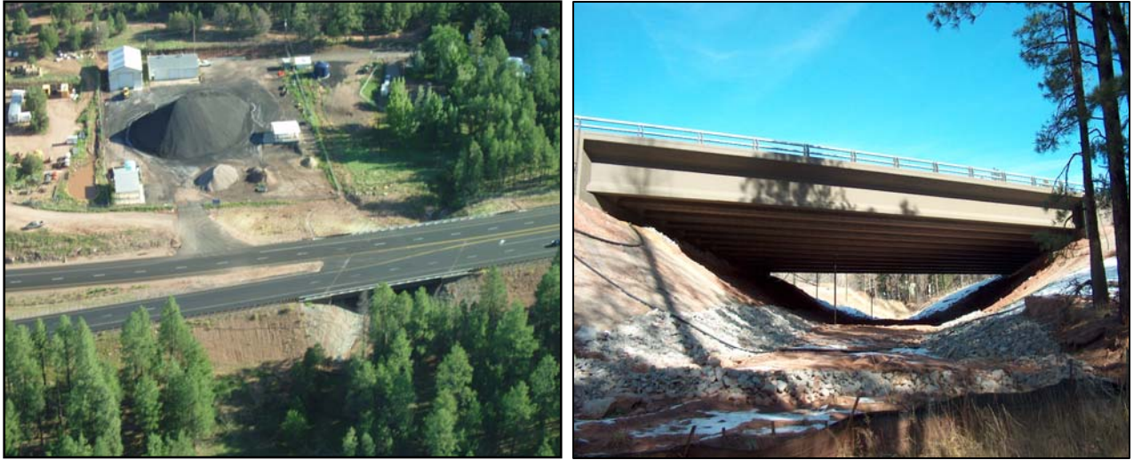
Figure 11.5. Aerial (left) and entry (right) views of the Wildlife 3 underpass looking north. Note that this is the only single-bridge underpass without an atrium that we monitored. Also note its proximity to the ADOT Colcord maintenance yard and residences (left).
