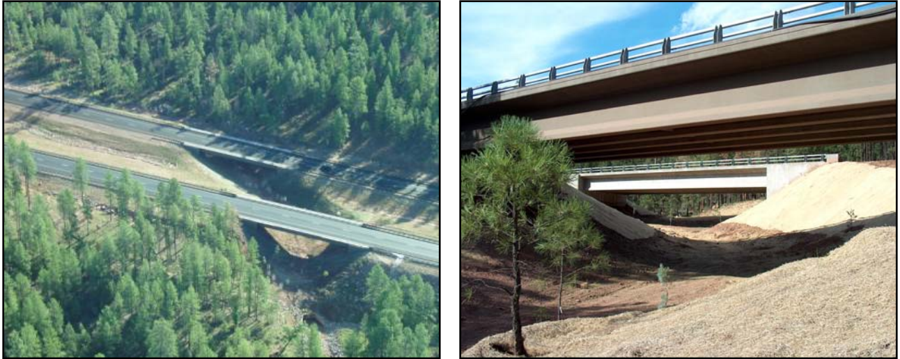
Figure 11.4. Aerial (left) and entry (right) views of the Wildlife 2 underpass looking north. Note how the underpass connects ponderosa pine forest on both sides of the highway and its wide atrium between bridges (left), as well as the relatively poor visibility through the underpass from the floor (right) associated with the offset nature of the bridge placement (left).
