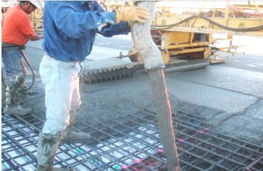
Figure 10. Pumping Concrete Using an “S” Pipe
