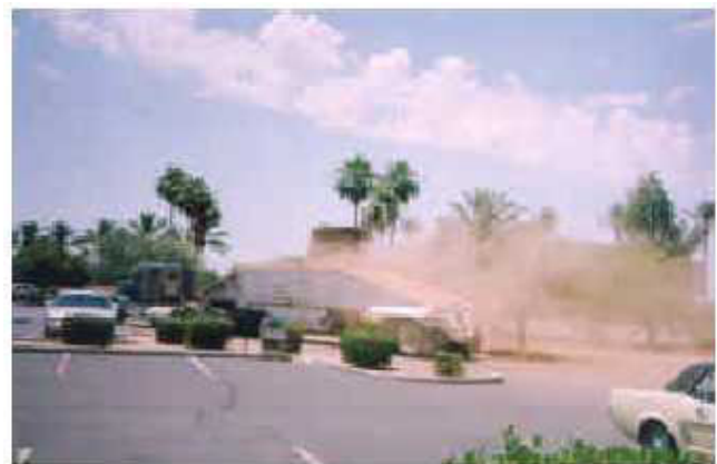
Uncovered loads of earth will create dust during hauling.
