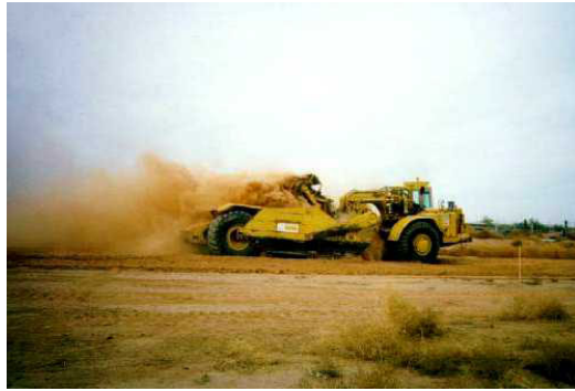
Earthmoving operations in dry soil can generate significant amounts of airborne dust.
