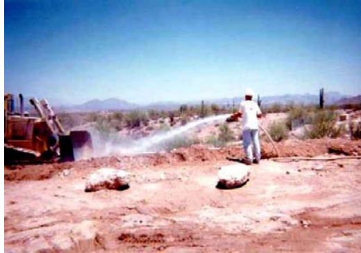
During trenching, water using a fine spray or mist.
