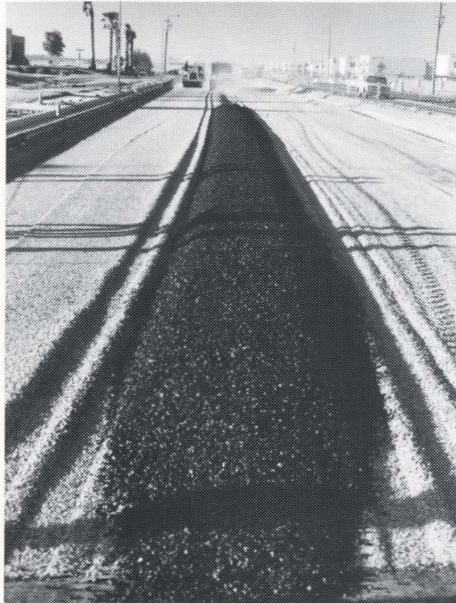
FIGURE 8 ASPHALT TREATED BASE COURSE SPREAD
