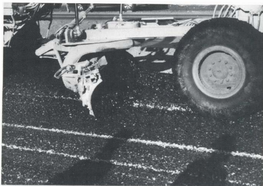
FIGURE 9 MOTOR GRADER PLACING FIRST LIFT OF OPEN-GRADED ASPHALT TREATED BASE COURSE
