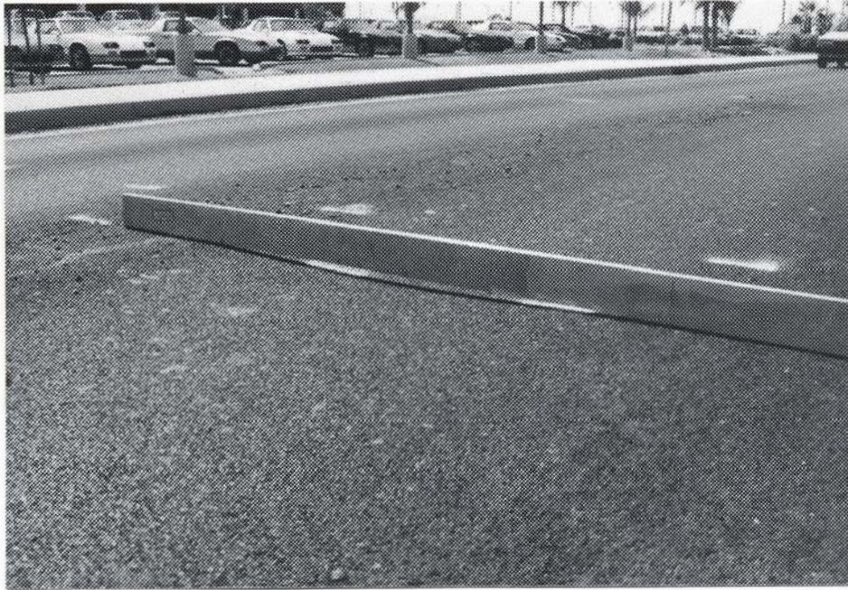
FIGURE 11 PAVEMENT DEFORMATION AT STATION 107 RT
