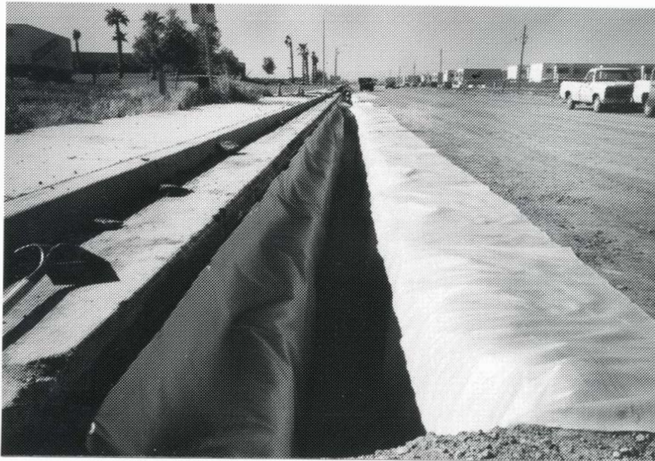
FIGURE 4 DRAINAGE TRENCH WITH FILTER FABRIC IN PLACE
