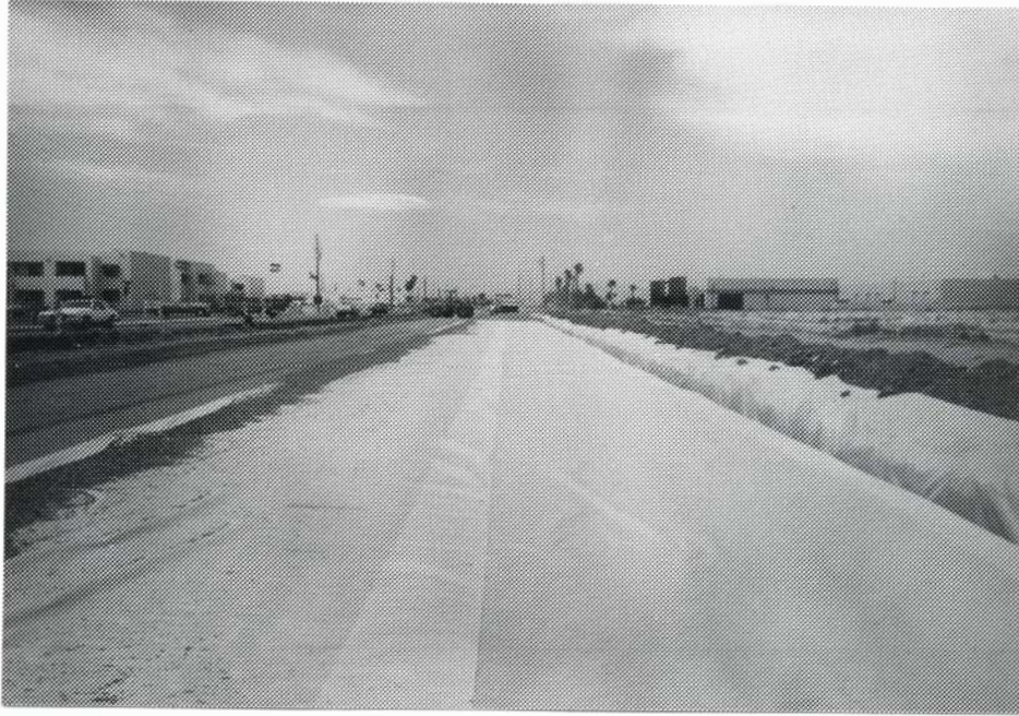
FIGURE 3 FILTER FABRIC IN PLACE
