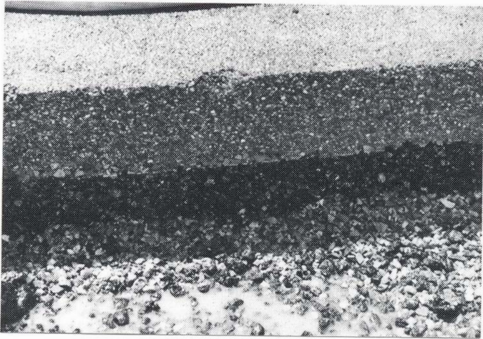
FIGURE 12 EXPOSED PAVEMENT LAYERS AT STATION 107 RT
