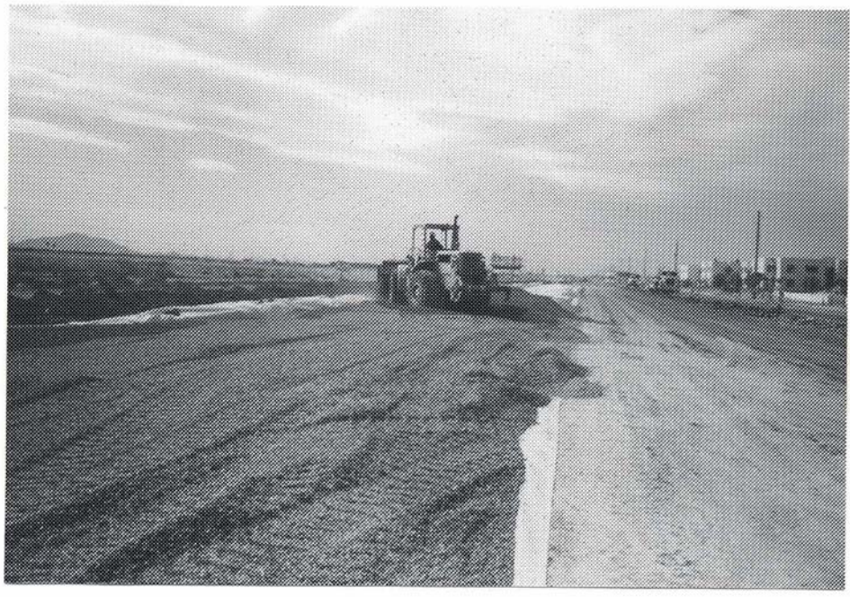
FIGURE 5 PLACING AND LEVELING OPEN-GRADED AGGREGATE SUBBASE
